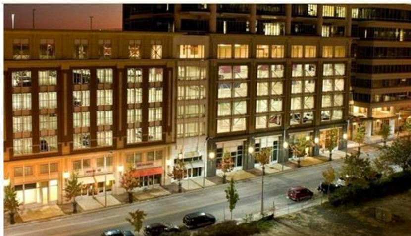
Block 100, E. Davie Street, Raleigh, N.C., with LED Lighting
