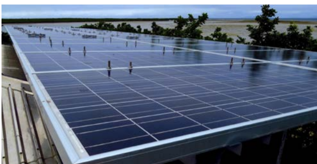
© Great Barrier Reef Marine Park Authority. Solar array 30 x 170W PV modules.
