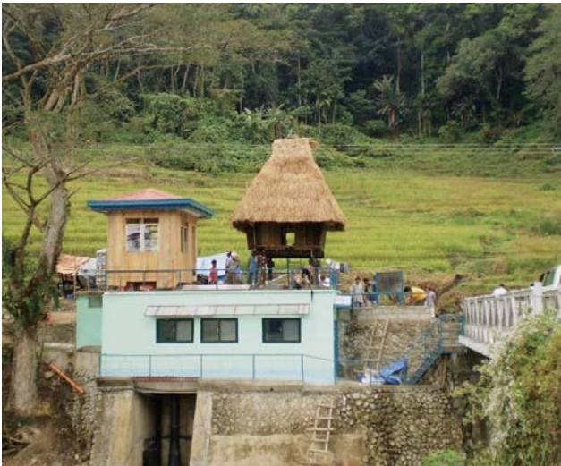
© Global Sustainable Electricity Partnership. Mini-hydro plant.
