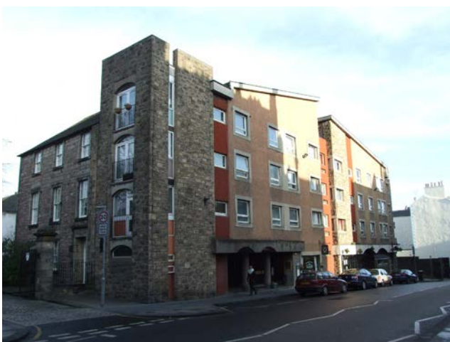
© EWH. Energy Efficiency for Post-War Listed Buildings.
