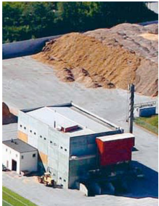
District heating plant in Visby
