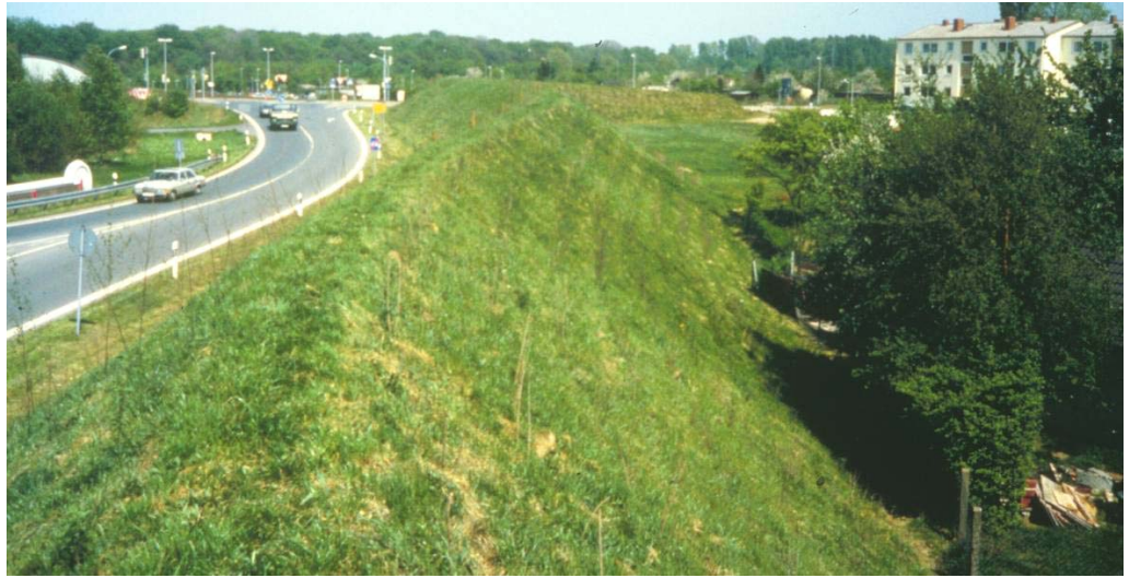
Figure 3.20. Earth embankment as a noise barrier in Germany.
