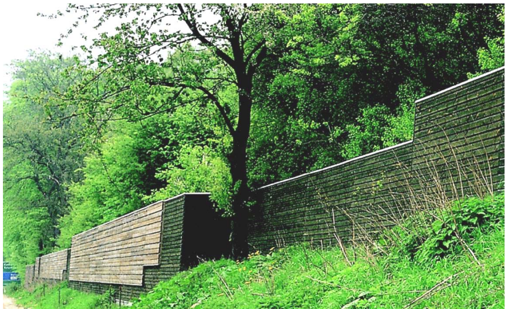
Figure 3.7. 3 m (10 ft) high wood noise barrier along a highway at the countryside adapted to the existing old vegetation at Highway M40 near Nyborg, Denmark [1].
