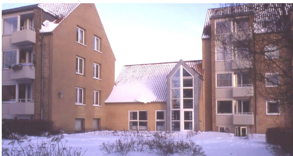
Figure 3.16. Two stories building with laundry and meeting room constructed between two apartment blocks also to function as a noise barrier for the road noise in the hole between the apartment blocks reducing the noise at the outdoor areas in Århus, Denmark.
