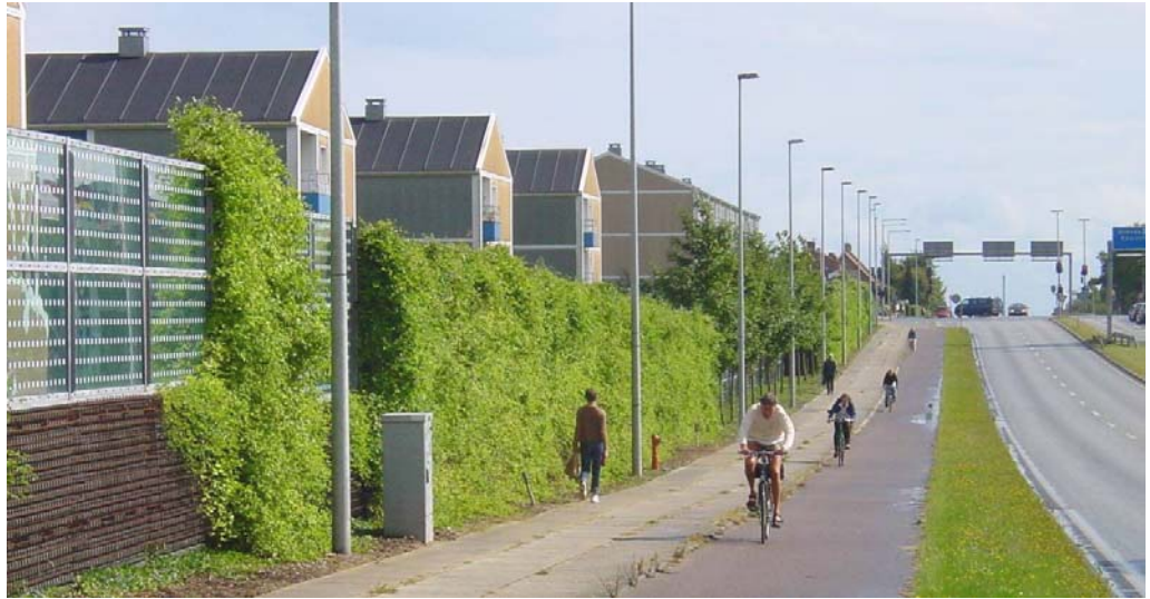
Figure 2.11. Danish transparent noise barrier with vegetation that can reduce the noise reflection.
