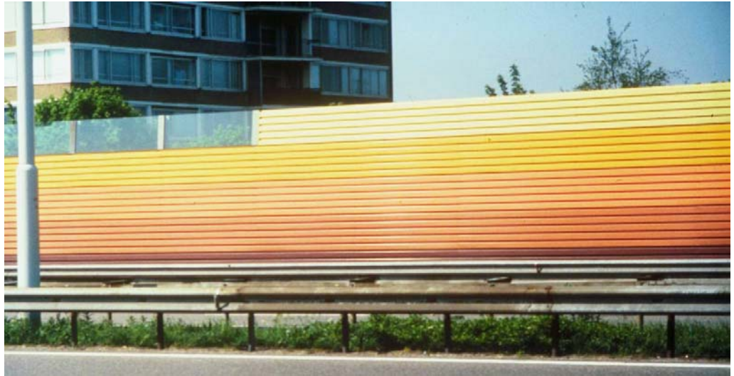
Figure 2.17. 4½ m high colored noise absorbing steel barrier with perforated surface and absorbing material at Highway A9 in the Netherlands [3].
