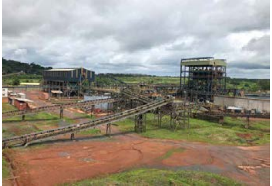
Partial view of the Marampa processing facilities, which have been well maintained through a care and maintenance programme implemented by Gerald, despite the harsh environment
