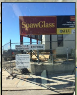
Construction of new Confluence Park
