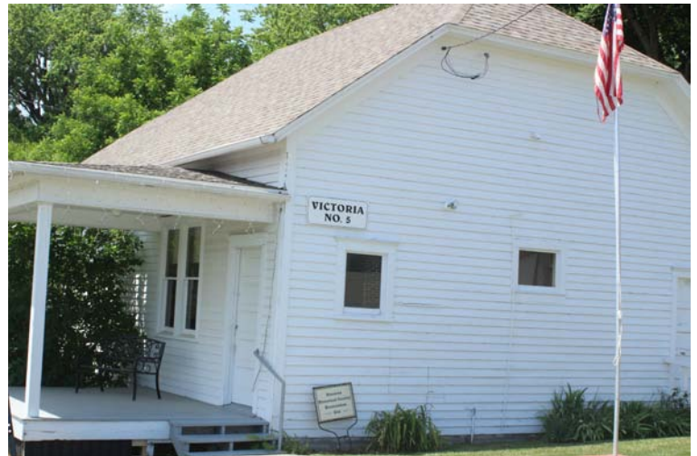
Massena One Room School House
