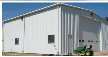
Addition to Existing Building
