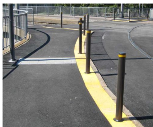
Figure 115: Pedestrian paths and platform edge marked with clear contrast (Source: Landskapsgruppen AB, Emma Johansson eller Roland Ahlgren där ej annat anges)
