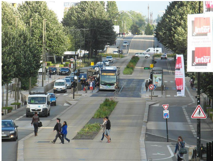
Figure 22: France Le Busway, Station overview (Source: https://commons.wikimedia.org/w/index.php?curid=22010918 )
