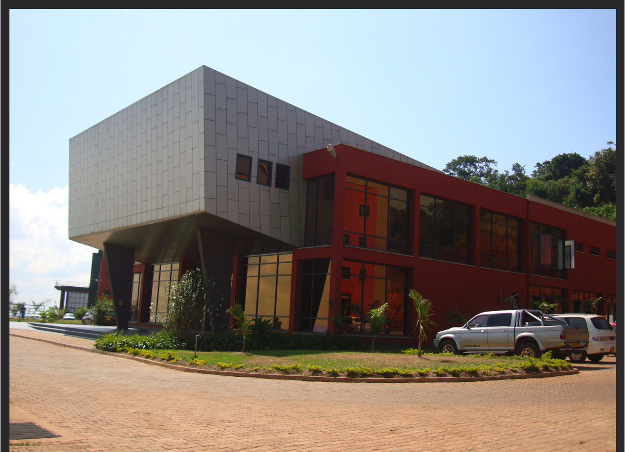
Chieftaincy of Military Intelligence building, Mbuya Hill, 2012. Photo obtained by Privacy International.
