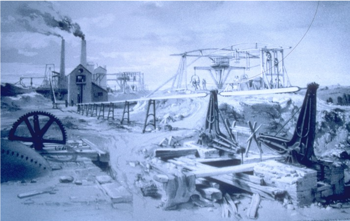
Fig. 5. Pumps for draining the Kilsby Tunnel (Bourne 1839: courtesy of the Institution of Civil Engineers Library)
