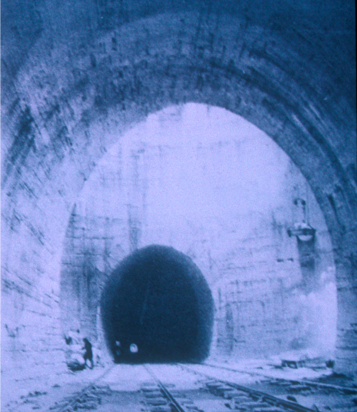
Fig. 2. Great ventilating shaft, Kilsby Tunnel (Bourne 1839: courtesy of the Institution of Civil Engineers Library)
