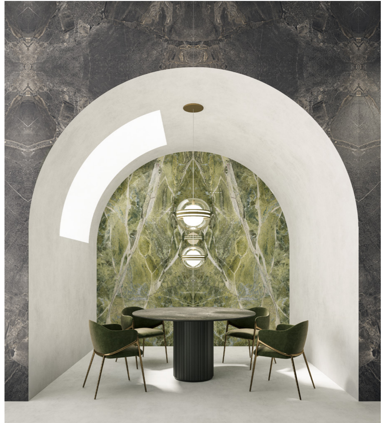
VERTICAL CLADDIED SURFACES PRE-CUT OFF-SITE (FIG.7.1)
