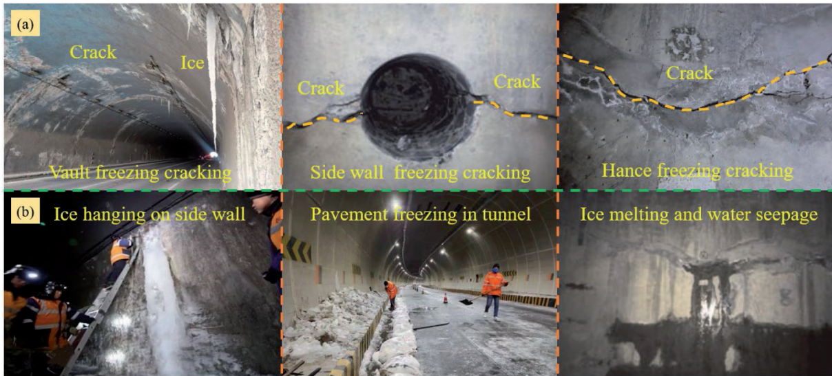
Fig. 14. Types of tunnel freezing damage: (a) structural freezing damage; (b) internal freezing damage [69, 70].
