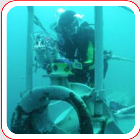
Principal Conservator Ian MacLeod, taking corrosion potential readings on the HMAS Perth.
