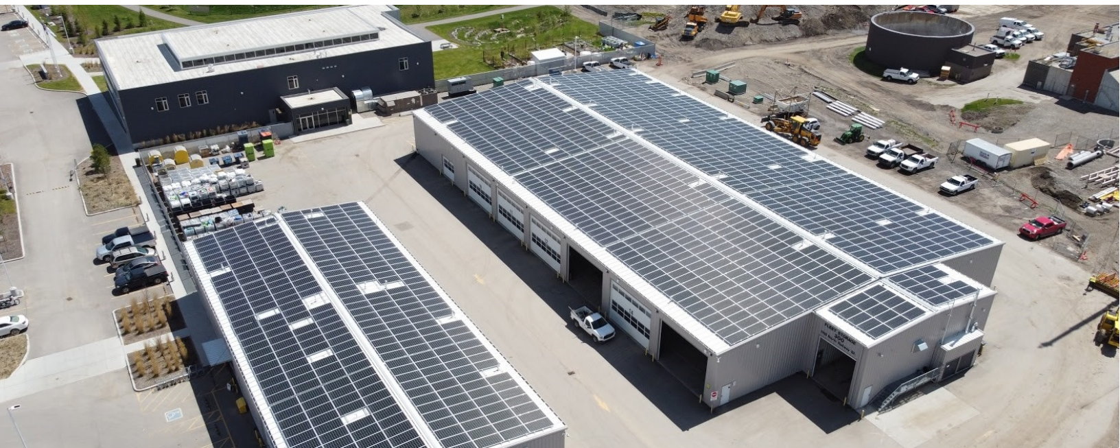
Solar PV System at the Operations Centre
