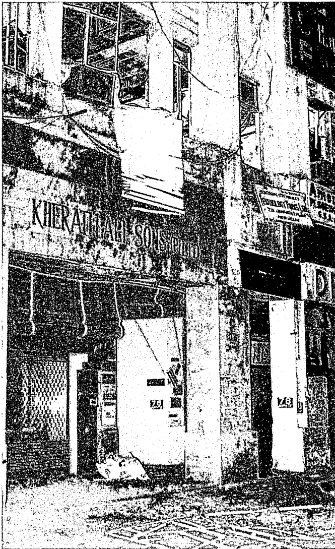
January 17, 1991—New Delhi, India: A powerful bomb exploded in the busy commercial area in Cannaught Place. Five rooms belonging to two establishments, including the office of an airlines agent dealing in American air tickets, were extensively damaged.
