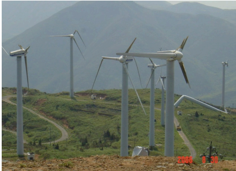
Picture 1: Vestas Turbines after a Typhoon
