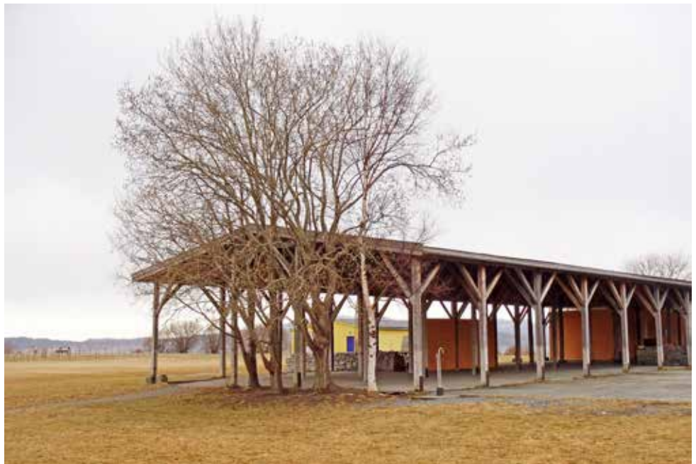
Figure 7.23 A military area was rearranged as a recreational area. Some buildings were allowed to remain; this one became a large outdoor barbecue site with a protective roof. A group of Salix caprea subsp. caprea (and one Betula pubescens ) were taken care of, probably to soften up the building.
