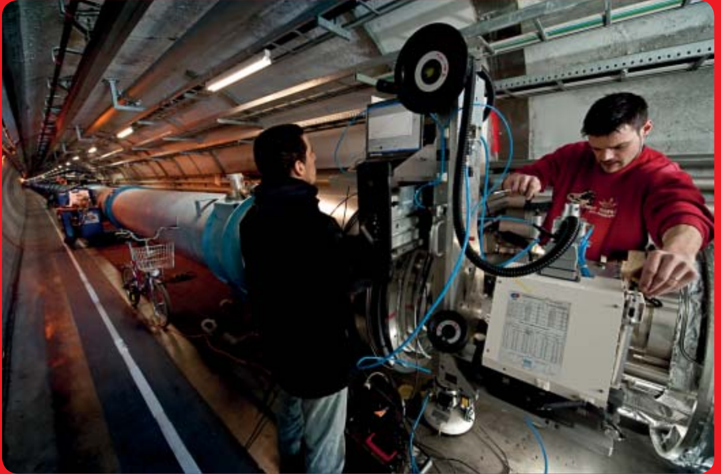
Figure 2.1.1. Welding of magnet interconnections during LHC repair in 2009.
