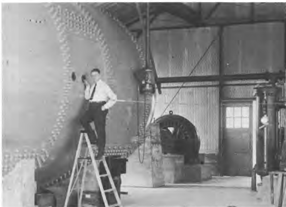
Max Munk in front of the variable-density wind tunnel that made his reputation, and the NACA's. (LaRC)
