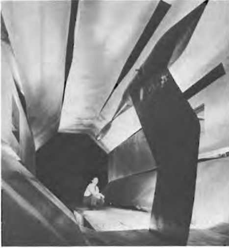
Left, a worker examines a model in the test section of Langley's 16-foot high-speed wind tunnel in 1951, shortly after the tunnel was repowered and equipped with the new slotted throat that reduced wall effects and permitted accurate testing in the anomalous transonic region around mach 1. Right, two workers survey the return passage of the same tunnel; the diameter here is 58 feet. (LaRC)
