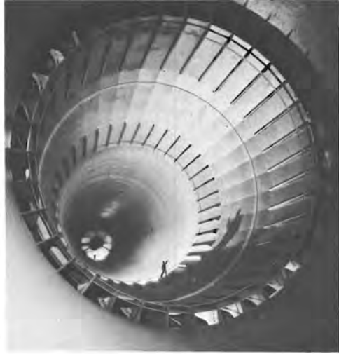
Left, a worker examines a model in the test section of Langley's 16-foot high-speed wind tunnel in 1951, shortly after the tunnel was repowered and equipped with the new slotted throat that reduced wall effects and permitted accurate testing in the anomalous transonic region around mach 1. Right, two workers survey the return passage of the same tunnel; the diameter here is 58 feet. (LaRC)
