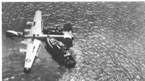
One of the NACA's more dramatic flight-research projects was the ditching test of a B-24 in the James River in 1944. The military services were greatly concerned at the time with the safety of crews in planes forced down over water. (LaRC)
