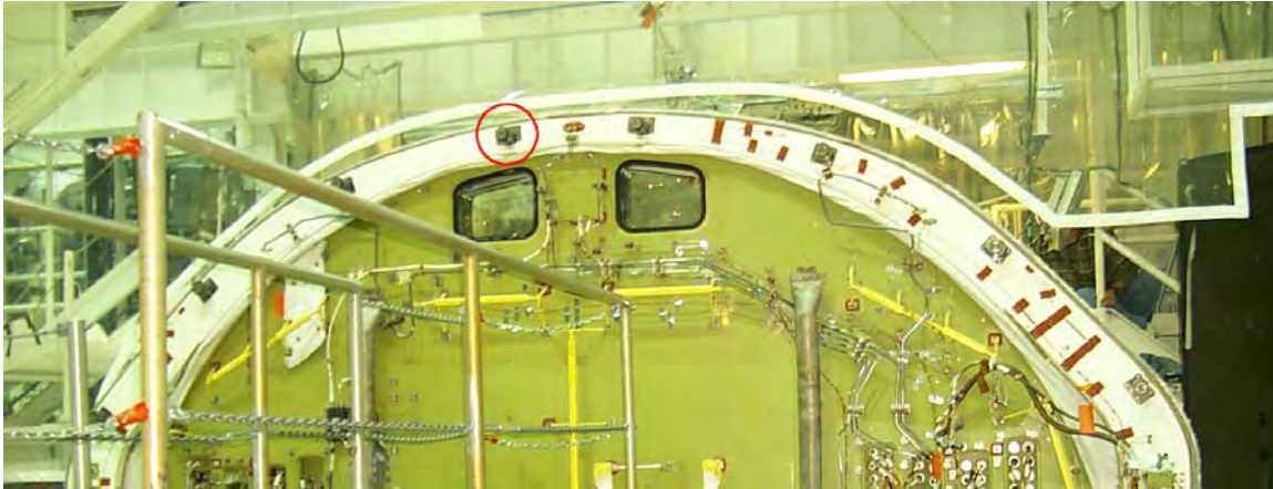
Figure 2.4-61. Endeavour, OV-105, X, 582 ring frame bulkhead arch with rollers. Circled in red is one of the eight rollers.
