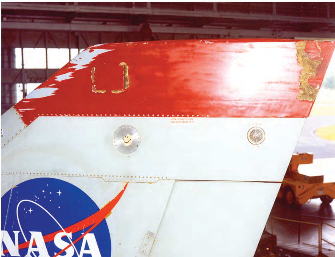
Damage to composite fin cap on F-106B. Note burn areas around inspection panel and near trailing edge of cap.
