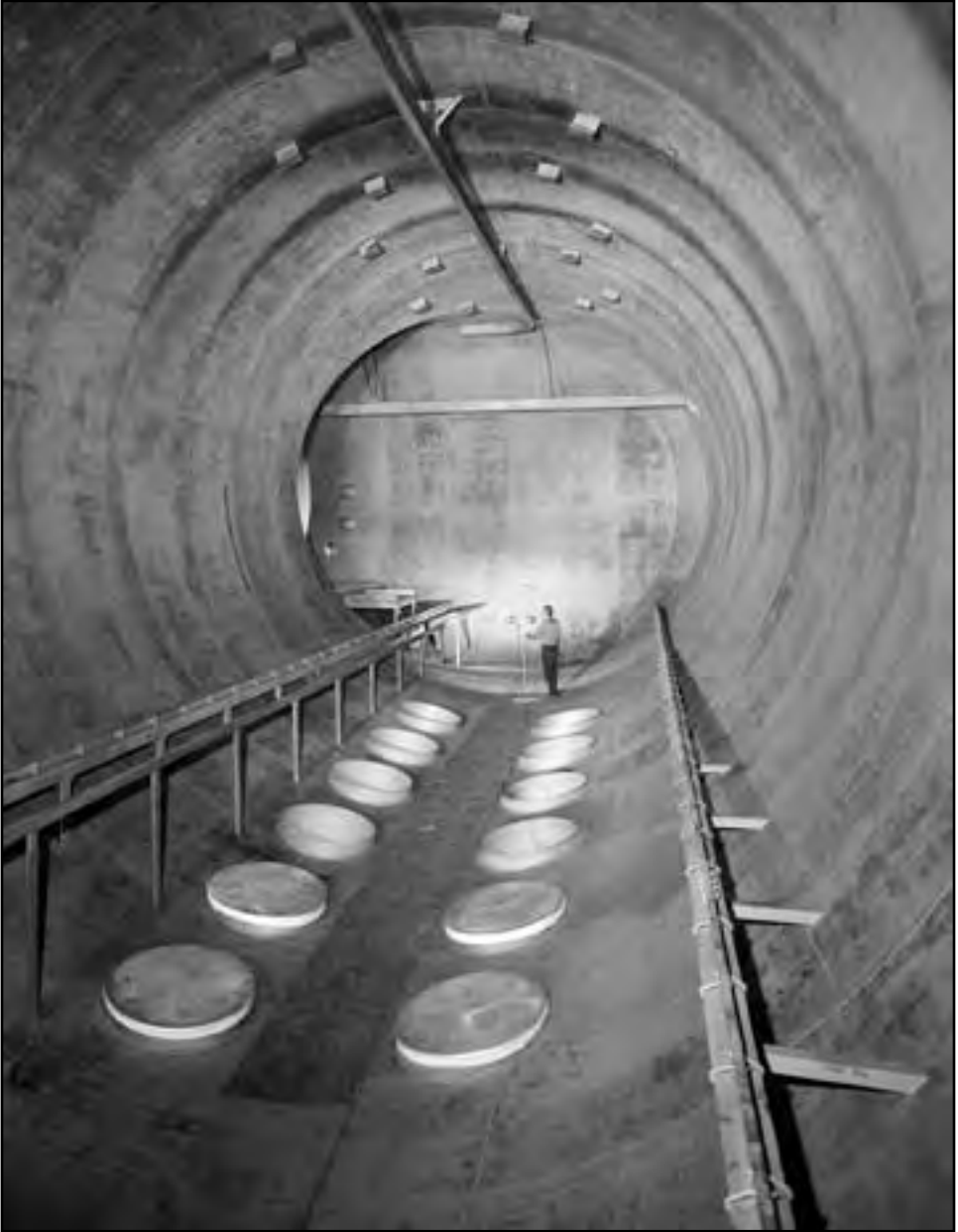
Image 186: SPC No. 1 in its initial configuration in the east leg of the tunnel. The 100-foot-long chamber was 31 feet in diameter at the southeast end, 27 feet in diameter at the northeast end, and had an internal volume of 70,000 cubic feet. 390 The diffusion pumps could reduce the atmosphere to a pressure level of 10^{-5} millimeters of mercury or roughly that found at an altitude of 100 miles. A removable dome would be added in the ceiling to lower a second-stage rocket into the tank. (NASA C-1962-61467)
