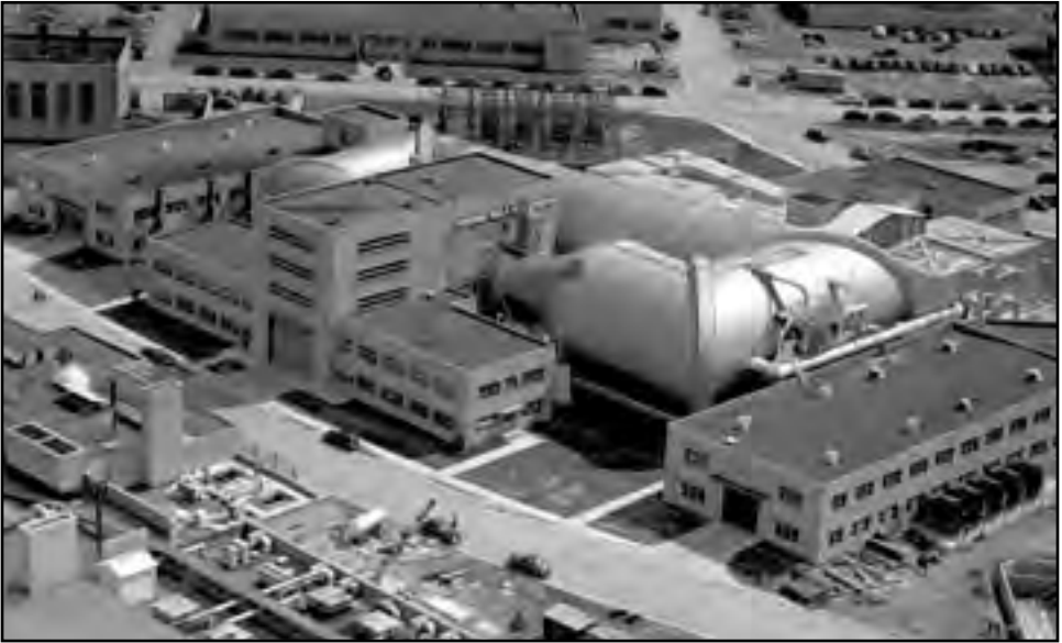
Image 39: The AWT complex as it originally appeared. The Shop and Office Building is in the center; the Refrigeration Building is to the right, and the Exhauster Building to the left. When completed in early 1944, it became the first wind tunnel in the nation designed specifically to study engine behavior and capable of creating a high-altitude environment. (NASA C-1945-13045).
