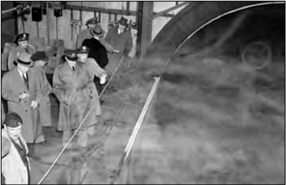
Image 61: NACA leaders accompany General Henry Arnold on his tour of the AWT on 9 November 1944. Here the group is on the tunnel's viewing platform peering into the 20-foot-diameter test section. The refrigerated air in the tunnel is vaporizing as it mixes with the warmer exterior air. Arnold pushed the development of jet engines during the war. This included the testing of nearly every early model in the AWT. (NASA C-1944-07499)
