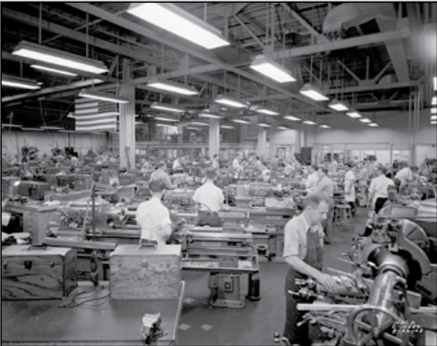
Image 52: Crowded conditions inside the Fabrication Shop. The lab was under pressure to meet the military's demand for wartime testing. This resulted in 48-hour weeks and three shifts per day. The AWT's late entry into the war left no time to spare. Those who were frequently absent or arrived late were transferred or discharged. 143 (NASA C-1945-10396)
