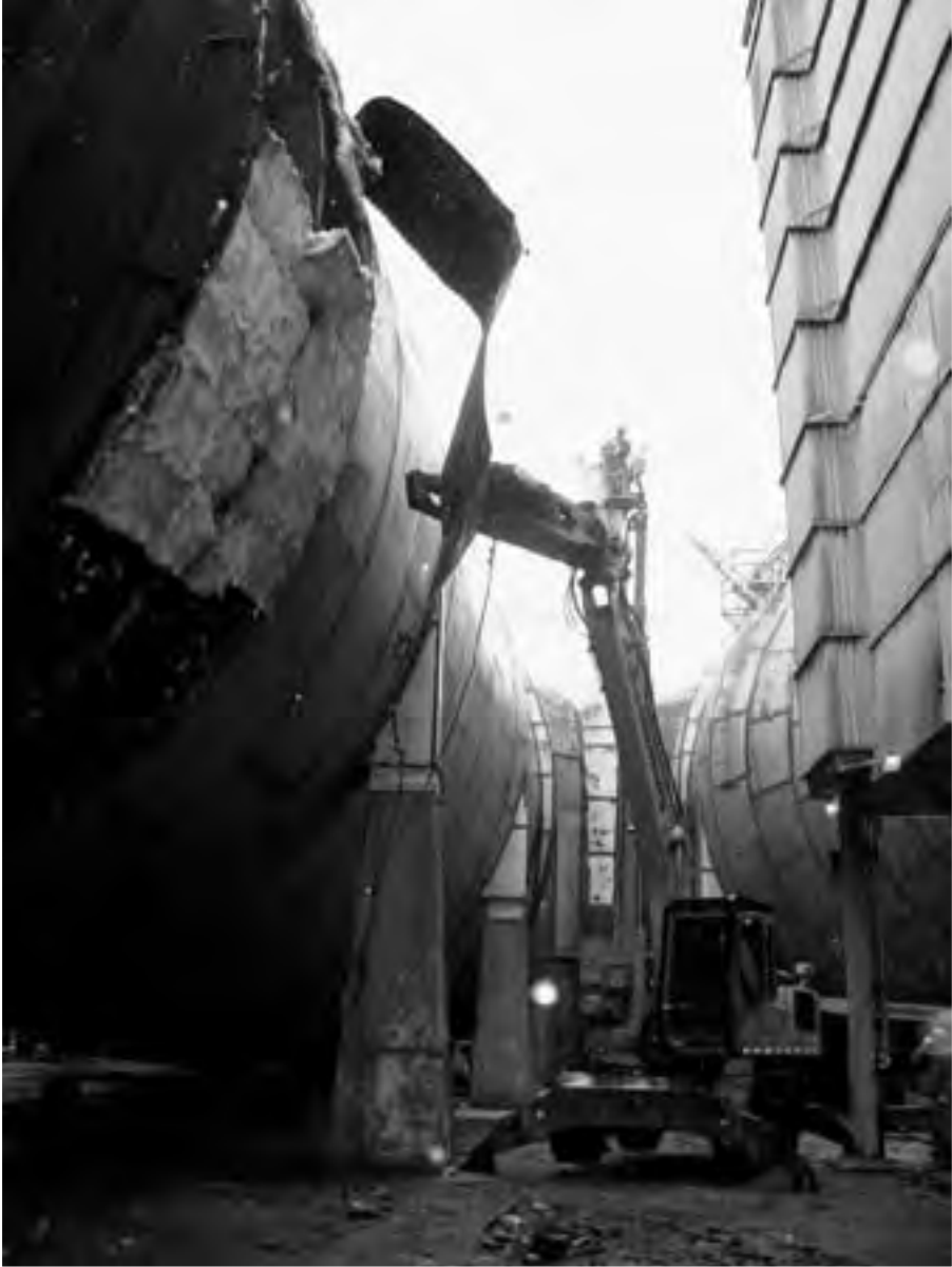
Image 283: Workers begin ripping off the outer shell. (NASA C-2008-04593)
