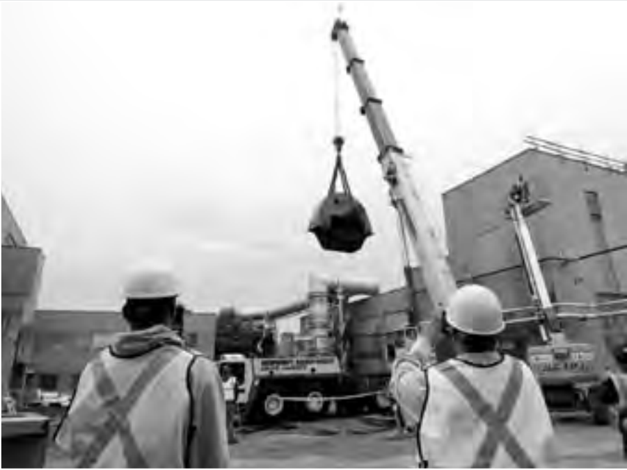
Image 288: One of the last tasks (1 June 2009) was lifting the drive motor out. (NASA G-2009-01589)
