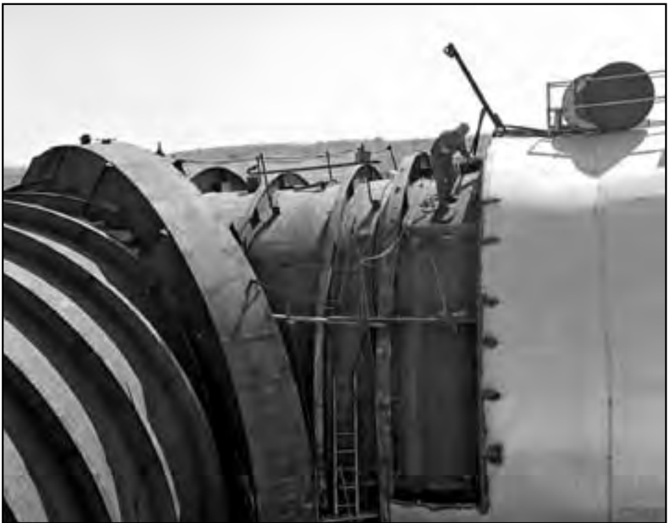
Image 178: A worker cuts away the AWT's outer shell in preparation for the installation of a large bulkhead and the sealing of the inner shell during the creation of the new SPC No.1 space tank. (NASA G-1961-58124)
