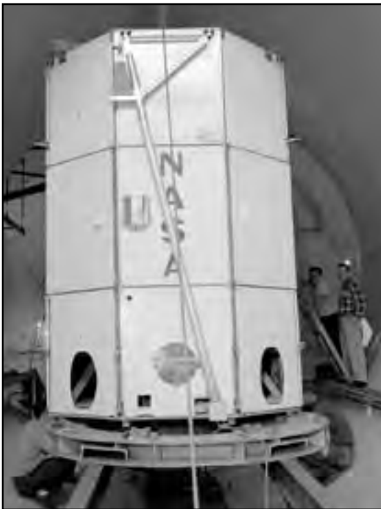
Image 244: A model of the OAO-2 observation satellite is transported through the former AWT test section and into SPC No. 2. OAO-2 contained two new experiments installed at opposite ends of the satellite. The Smithsonian Astrophysical Laboratory's experiment consisted of four telescopes capable of examining over 700 stars every day. The University of Wisconsin's study employed seven telescopes to study single stars for longer durations to determine the chemical composition, temperature, and pressure. 522 (NASA C-1968-01709)
