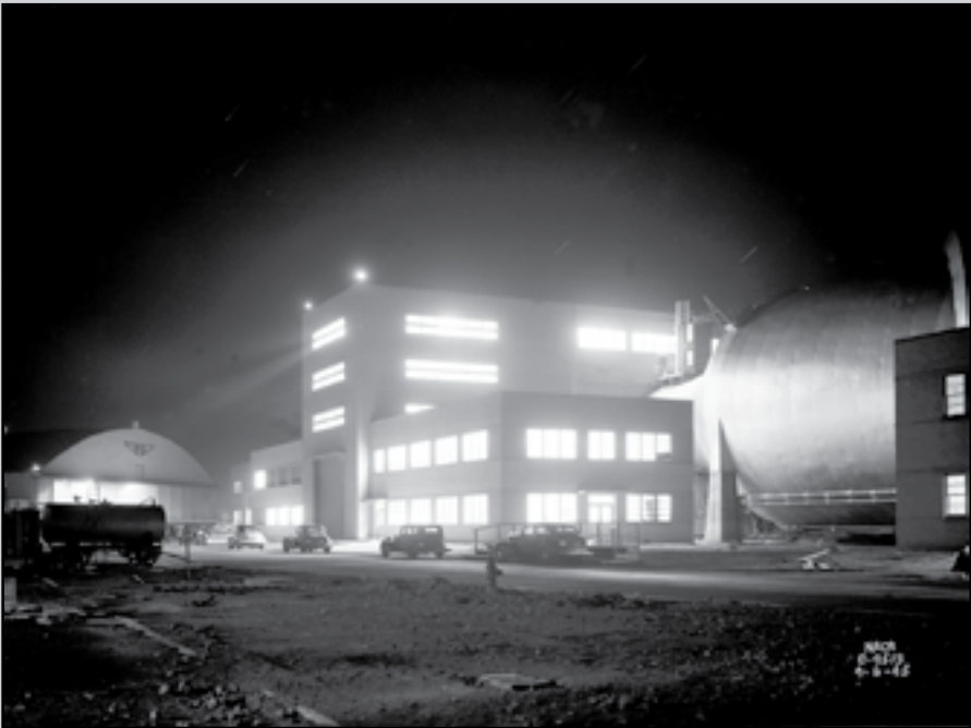
Image 51: The AWT seen during its overnight operation. The tunnel was usually run at night when the electric company had sufficient electricity for the massive power loads. (NASA C-1945-09513)
