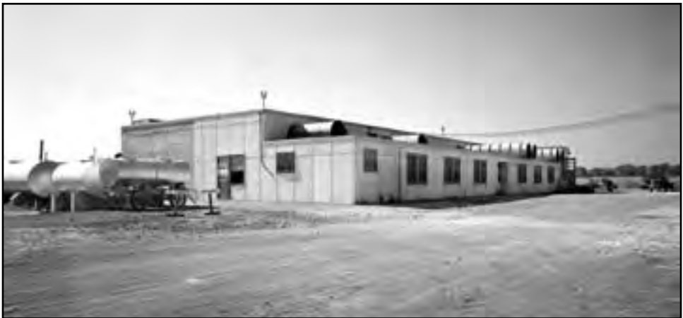
Image 45: Jet Propulsion Static Laboratory at the AERL. GE's West Lynn team had designed this nondescript two-cell test bed to be built at the AERL to test their new Whittle-based jet engines. An I-A, the first turbojet built in the United States, was secretly brought onto the lab disguised as a supercharger and tested in the Jet Propulsion Static Laboratory in the fall of 1943. The I-A had been superseded by the I-16 by this point. The I-16 would be tested in the AWT just a couple of months afterward. (NASA C-1945-12097)
