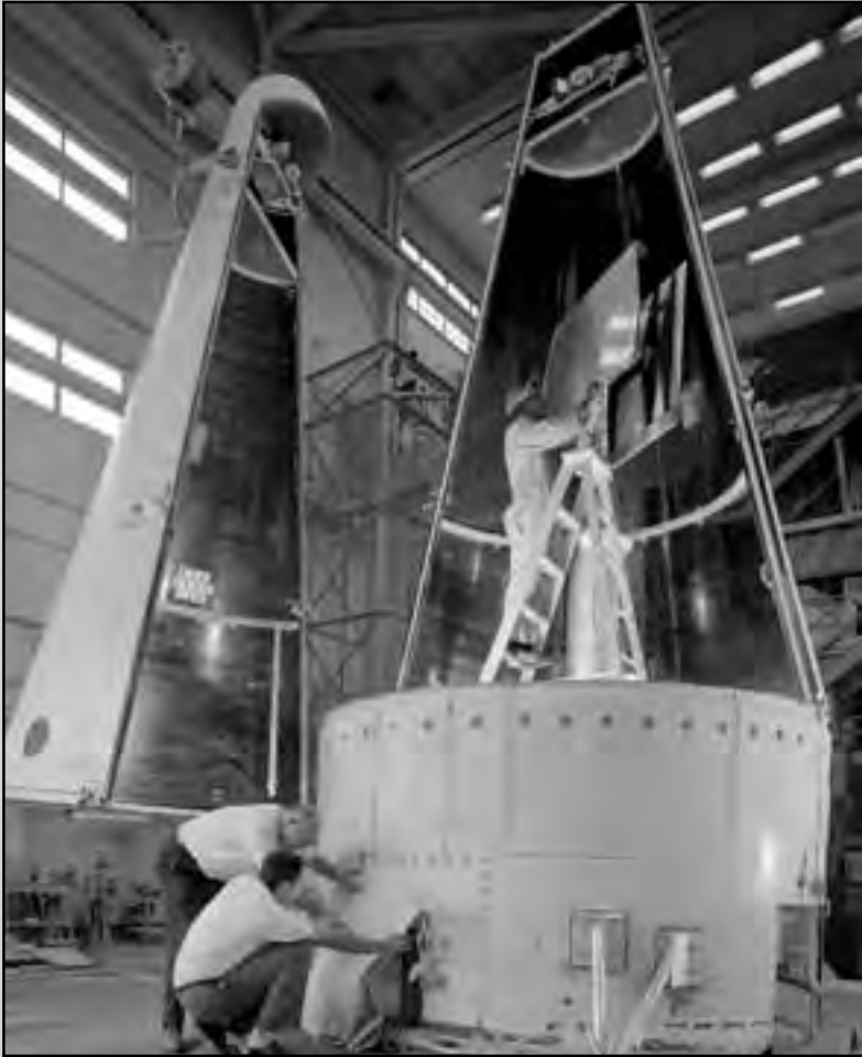
Image 206: As Lewis shifted from aeronautics research to spacecraft development work in the early 1960s, the center’s engineers and mechanics had to alter the way that they approached tests. Aircraft engines could often be tinkered with to improve performance, but space hardware required precision and adherence to specifications. Here a Surveyor nose cone is prepared in the high bay for separation tests in SPC No. 1. (NASA C-1964-70592)
