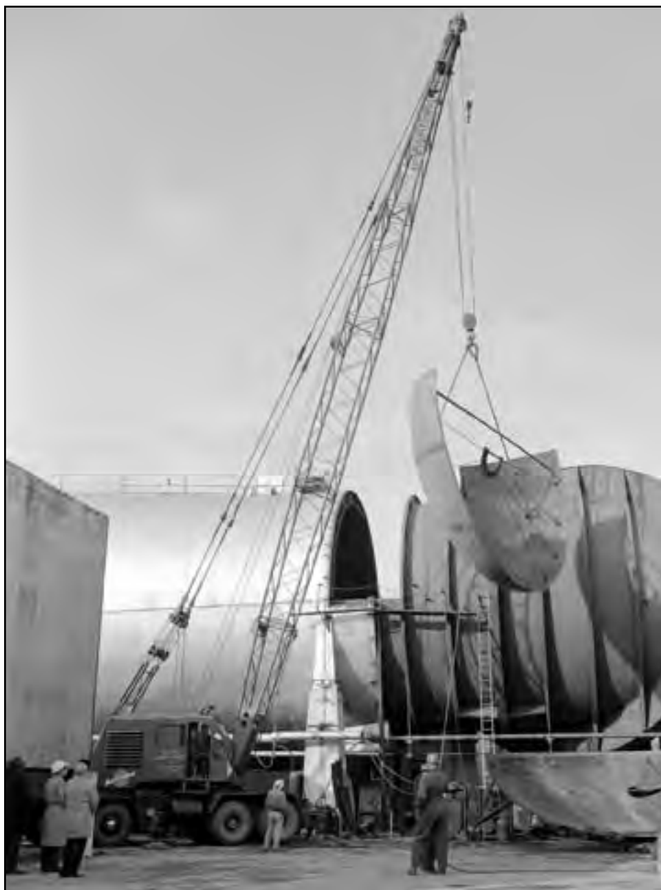
Image 172: Conversion of the Altitude Wind Tunnel into two altitude chambers. This photograph shows the largest of the three bulkheads being inserted into the tunnel. It is being placed approximately where the wind tunnel fan was located. (NASA C-1961-58551)
