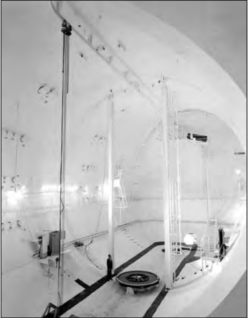
Image 187: SPC No. 2 in the western end and throat section of the tunnel. The section visible in this photograph was 51 feet in diameter and 121 feet long. The chamber also included the tunnel's throat section, which narrowed from 51 feet to 20 feet in diameter, and the back leg of the tunnel. The chamber used the existing tunnel exhaust systems to simulate altitudes of 100,000 feet. (NASA C-1965-00703)
