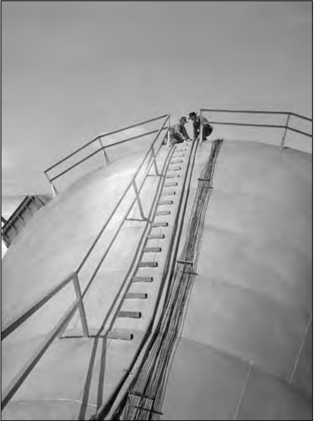
Image 76: Two men work on top of the 51-foot-diameter section of the Altitude Wind Tunnel. The facility emerged from the secrecy of the war and began a highly productive 10-year period of advancing turbojet technology. (NASA C-1945-10525)
