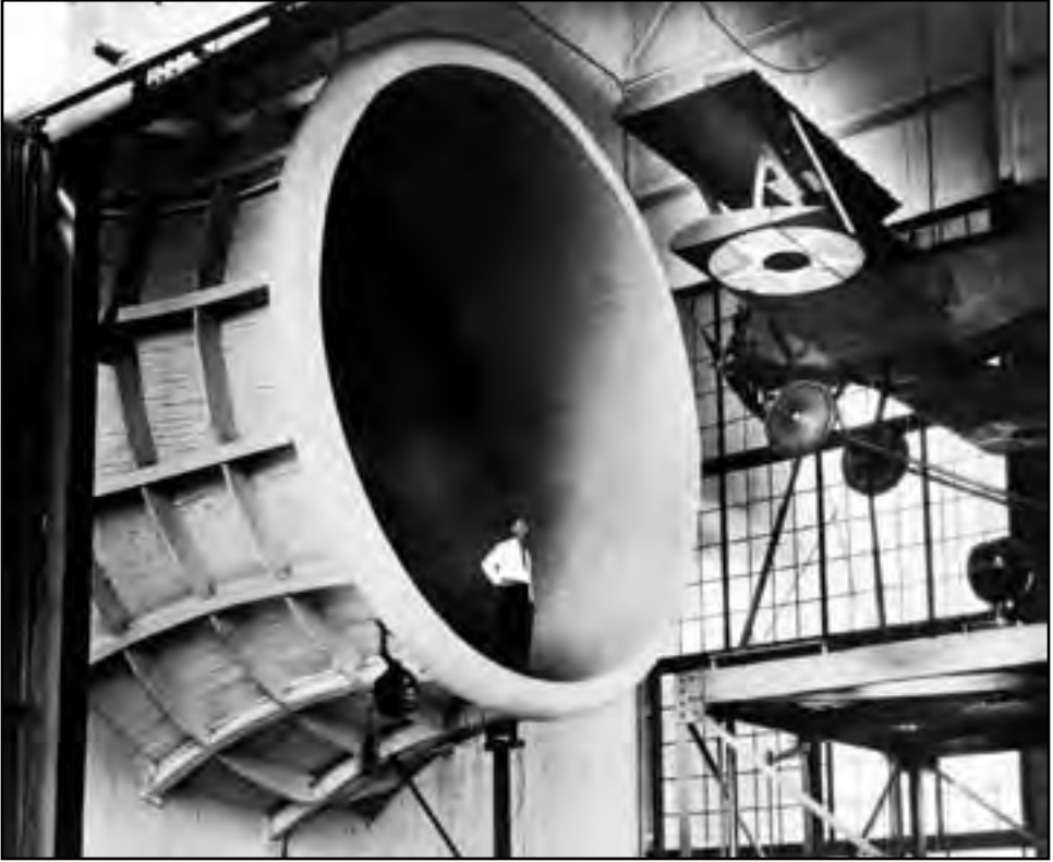
Image 7: Elton Miller, successor to Max Munk as Langley's chief of aerodynamics, stands in the exit cone of the Propeller Research Tunnel to view the Sperry M-1 Messenger during the tunnel's first runs. The Propeller Research Tunnel at Langley was used to clean up drag caused by aircraft engines but not to study the performance of those engines. The tests were run in atmospheric conditions and at relatively slow speeds. (1927) (NASA EL-01892)
