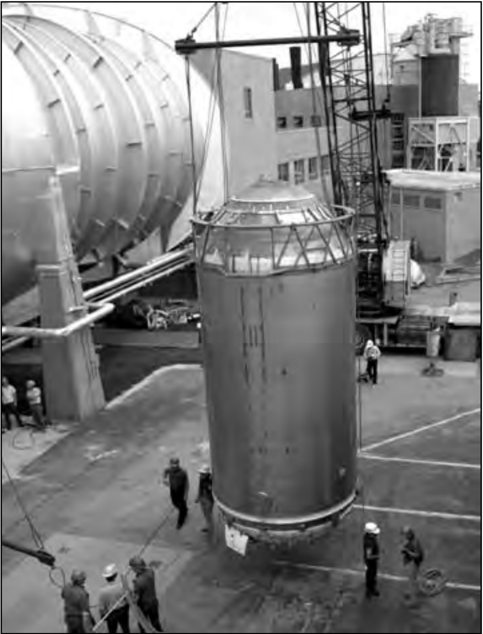
Image 264: A Centaur 6A rocket was placed inside SPC No. 1 in 1963 for long-duration space environment testing. Although the studies ended in the late 1960s, the rocket remained inside the chamber until August 1984. It was decided to remove the Centaur when the center considered returning the facility to its original wind tunnel configuration. (NASA G-1984-04470)
