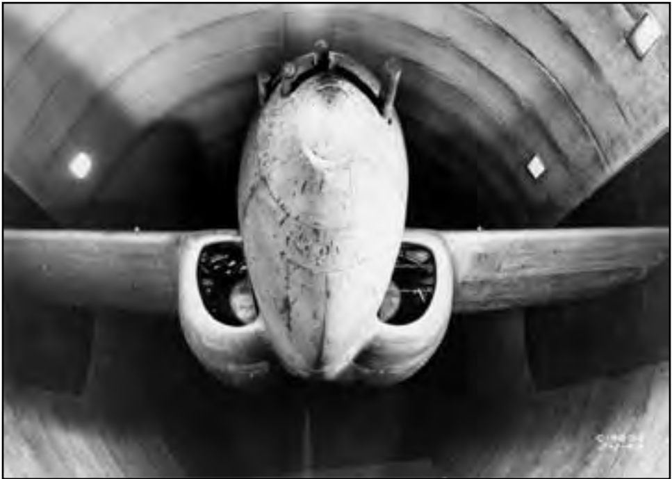
Image 47: The AWT's first test: the Bell YP-59A with its two GE I-16 turbojet engines. Improvements from the AWT tests included a boundary-layer removal duct, which decreased the fuselage's boundary layer by 60 percent; a new nacelle inlet, which in combination with the boundary-layer removal duct resulted in an additional 16-percent average pressure recovery near the compressor inlets; and new engine cooling seals, which reduced the nacelle's cooling airflow by 75 percent. 133 (NASA C-1944-04825)
