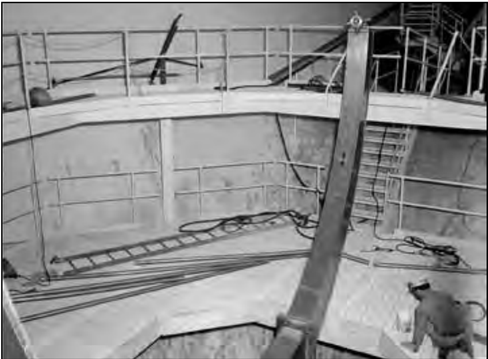
Image 153: Construction of the MASTIF inside the AWT to test the autopilot and attitude control systems for the Big Joe Mercury capsule. The MASTIF was built near the tunnel's throat section, with stairs installed to reach the test section and observation platform. (NASA C-1959-50266)
