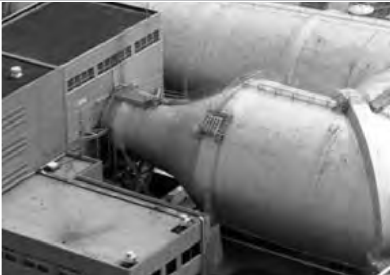
Image 102: The tunnel contracted just prior to the test section to increase the velocity of the airflow. This "throat" section narrowed from 51 to 20 feet in diameter. (NASA C-1979-04019)
