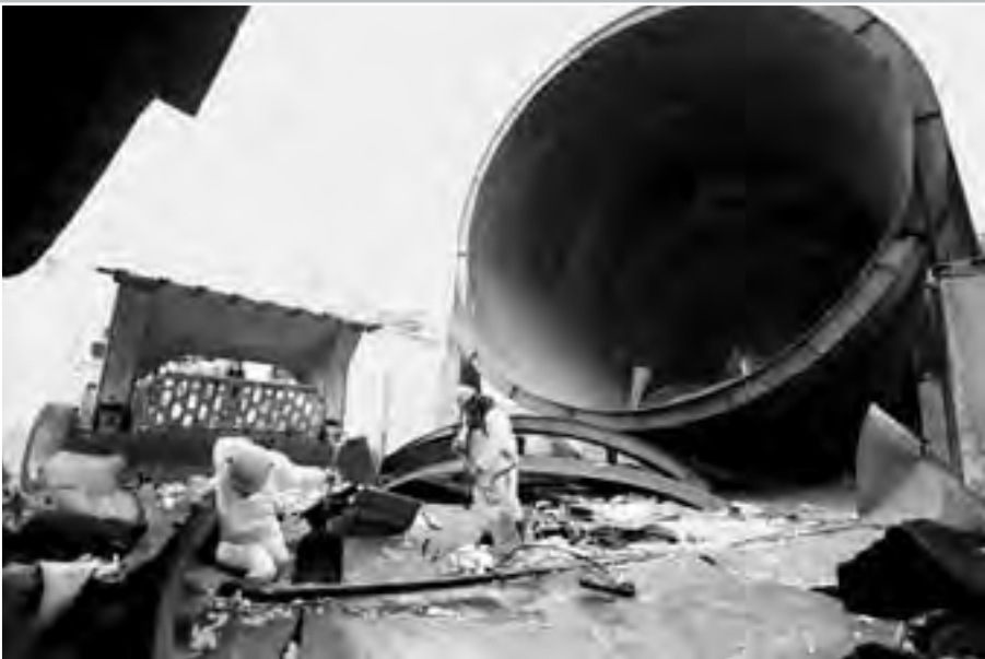
Image 289: Workers clean up debris at the AWT demolition site. (NASA G-2009-00100)
