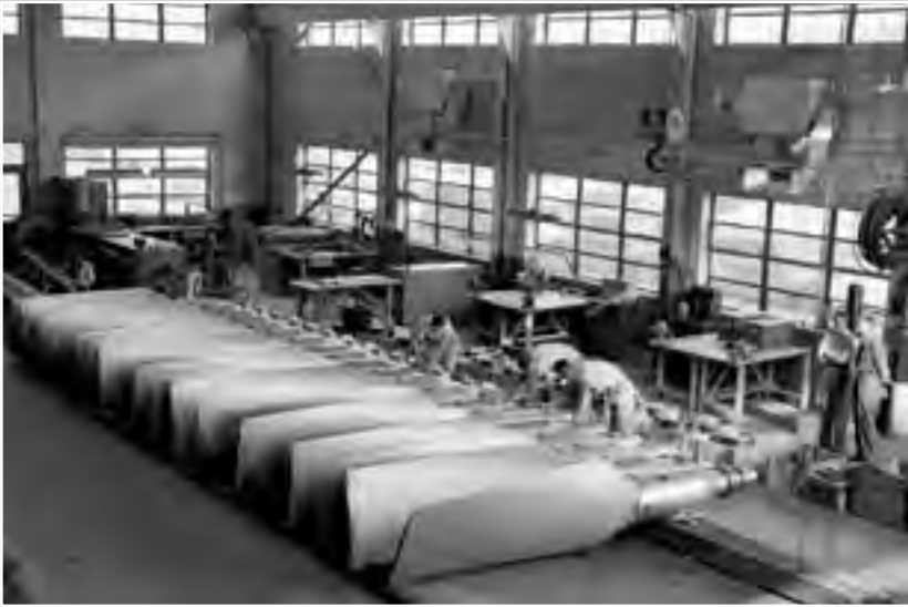
Image 126: The AWT's fan blades occasionally became worn or broken and had to be replaced. A new set of blades was installed on the 31-foot-diameter drive fan in 1951. The blades were prepared in the shop area, seen in this photograph, before being lowered into the AWT through a hole in the top of the tunnel and attached to the drive shaft. (NASA C-1951-28240)
