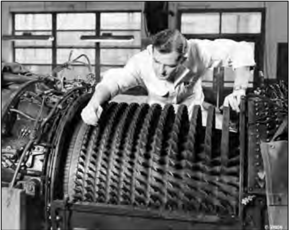
Image 115: A technician measures one of the TG-190 engine's stator blades. The GE TG-190 (J47) was a successor to the TG-180. A different 12-stage axial-flow compressor and a single-stage turbine were installed in the TG-180 frame. 255 The TG-190 went through numerous studies in the AWT during 1948 and 1949. (NASA C-1949-22850)
