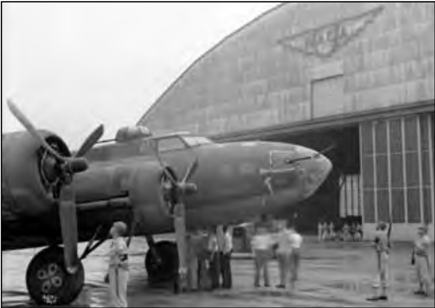
Image 27: On 7 July 1943 the Memphis Belle and its crew visited the AERL as part of a publicity tour. The B-17 Flying Fortress and its crew were returning after 25 successful bombing missions over Germany. Inside the hangar in the background, the large fan for the AWT was being assembled at the time. (NASA C-1943-1867)
