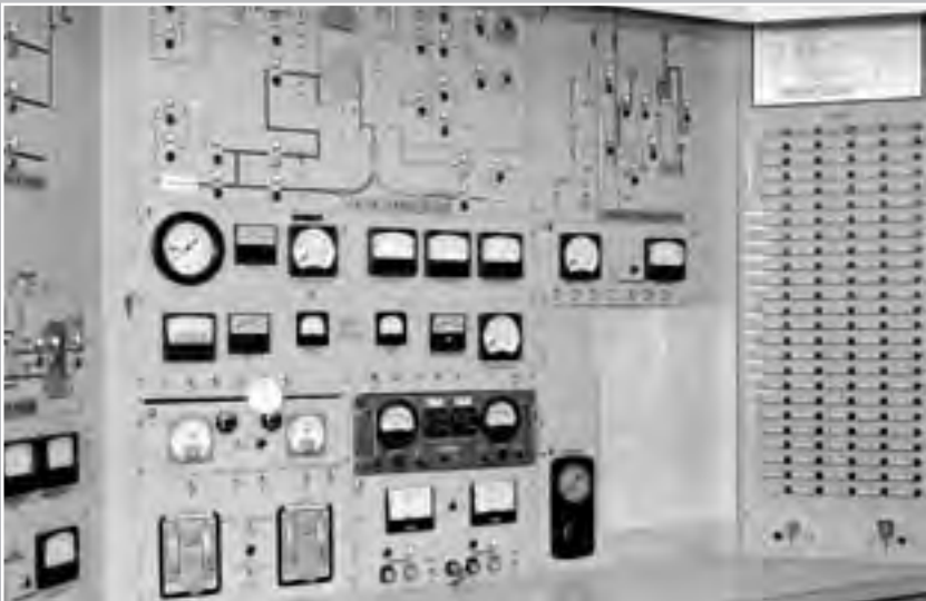
Image 216: The SPC No. 1 control room was constructed underneath the former wind tunnel test section. It was built to replicate the Centaur controls at Cape Canaveral. This panel operated the tanking system for the Centaur 6A rocket in the vacuum chamber. There was extensive instrumentation for the tests, including 200 transducers, 18 landlines, and a television camera. (NASA G-1967-00193)
