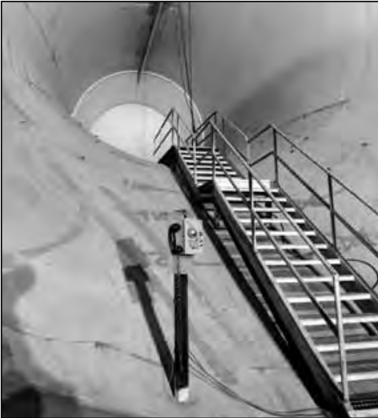
Image 270: Throat section of the AWT as seen on 5 April 2005 during a photographic survey prior to the tunnel's demolition. The stairs and telephone were installed for the Project Mercury tests in the late 1950s, including the Multi-Axis Space Test Inertia Facility (MASTIF). A bulkhead sealed the leg off from the former test section on the other side. (NASA C-2007-00377)
