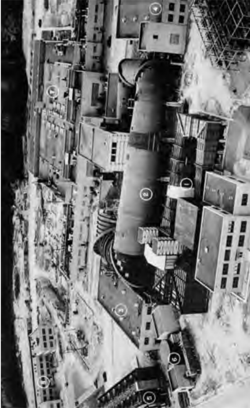
Image 86: The AWT complex, seen here with 1) the Icing Research Tunnel, included a number of support buildings; 2) the AWT, 3) the Refrigeration Building, 4) the Exhauster Building, 5) Cooling Tower No. 1, and 6) the Air Dryer Building. (NASA C-1944-05062)
