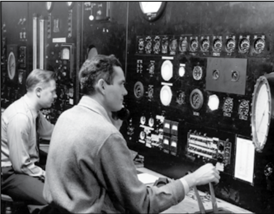
Image 67: Left to right: Roger Weining and Bob Godman operate an engine from the AWT's control room. The tunnel's ability to repeatedly study a full-size engine under flight conditions and engine parameters of their choosing allowed the researchers to make modifications and test them quickly without the expense and uncontrolled variables of flight testing. (NASA C-1945-10365)
