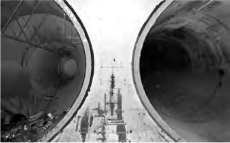
Image 274: Interior of the AWT/SPC as it appeared in 2005. The section to the left, where the MASTIF had been set up 45 years before, was later used to store holiday decorations (viewed from the west). (NASA C-2005-01615)
