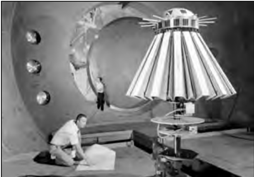
Image 174: Meteor Impact Model in the new SPC No. 1. This satellite was set up in the chamber days after the facility was officially rededicated as the Space Power Chambers (SPC) on 12 September 1962. The space tank was envisioned for the study of small satellites like this one. (18 Sept. 1962) (NASA C-1962-61717)
