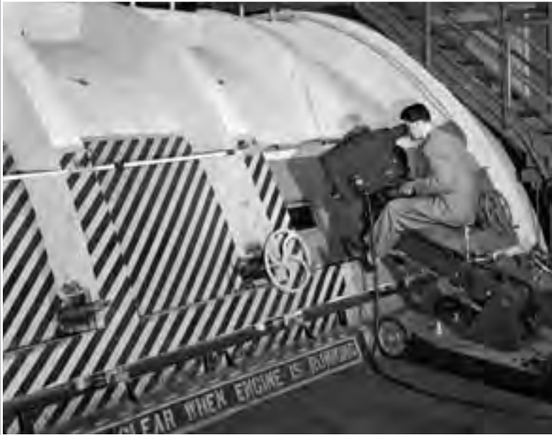
Image 93: The tunnel's clamshell lid was then lowered and fastened into place using hand-turned locking wheels. Windows along the side of the lid allowed photographers to film the test and observers to watch for engine failures. (NASA C-1951-28499)
