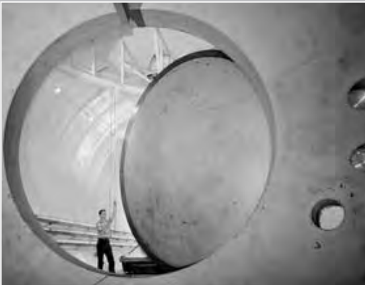
Image 183: Twenty-seven-foot-diameter bulkhead at the north end of SPC No. 1. It contained a swinging 15-foot-diameter door in the middle that permitted the movement of large articles into and out of the chamber. (NASA C-1962-61466)
