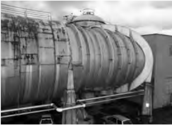
Image 271: Exterior of SPC No. 1 in 2005. The inner tunnel shell was in relatively good shape, but the exterior weather shell, seen to the left, was heavily rusted. (NASA C-2005-01670)
