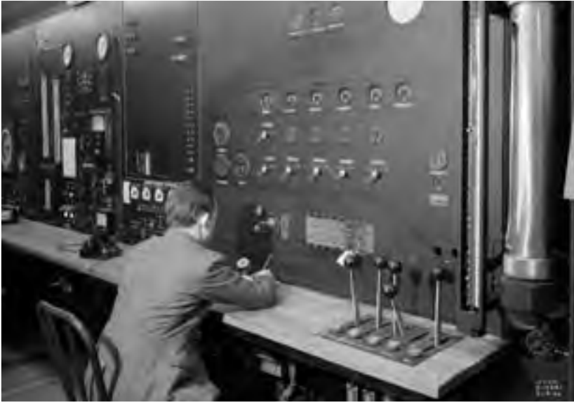
Image 105: The researcher at this station in the control room controlled the engine in the test section. The soundproof control room was located in the balance chamber next to the lower portion of the test section. From here the researcher could run the engine at various power levels and monitor numerous aspects of the engine's behavior. (NASA C-1946-14241)
