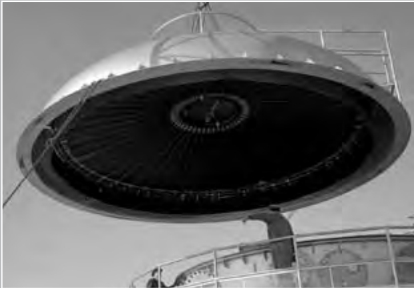
Image 212: The 22.5-foot-diameter dome being placed onto SPC No. 1. Instrument portals can be seen at the fixed-base of the dome. The top of the ribbed cold wall is visible inside the lid. (NASA C-1964-67913)
