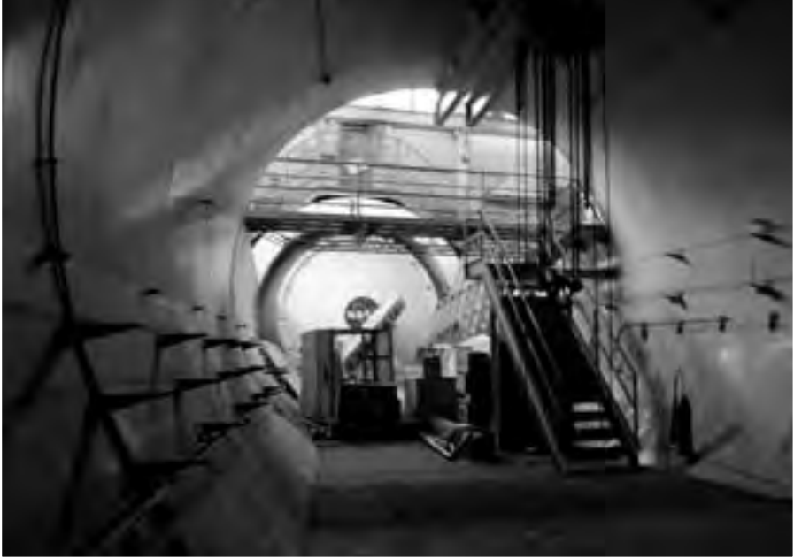
Image 276: View into the former test section. The area had been used to store large antenna equipment in recent years. (NASA C-2009-00763)
