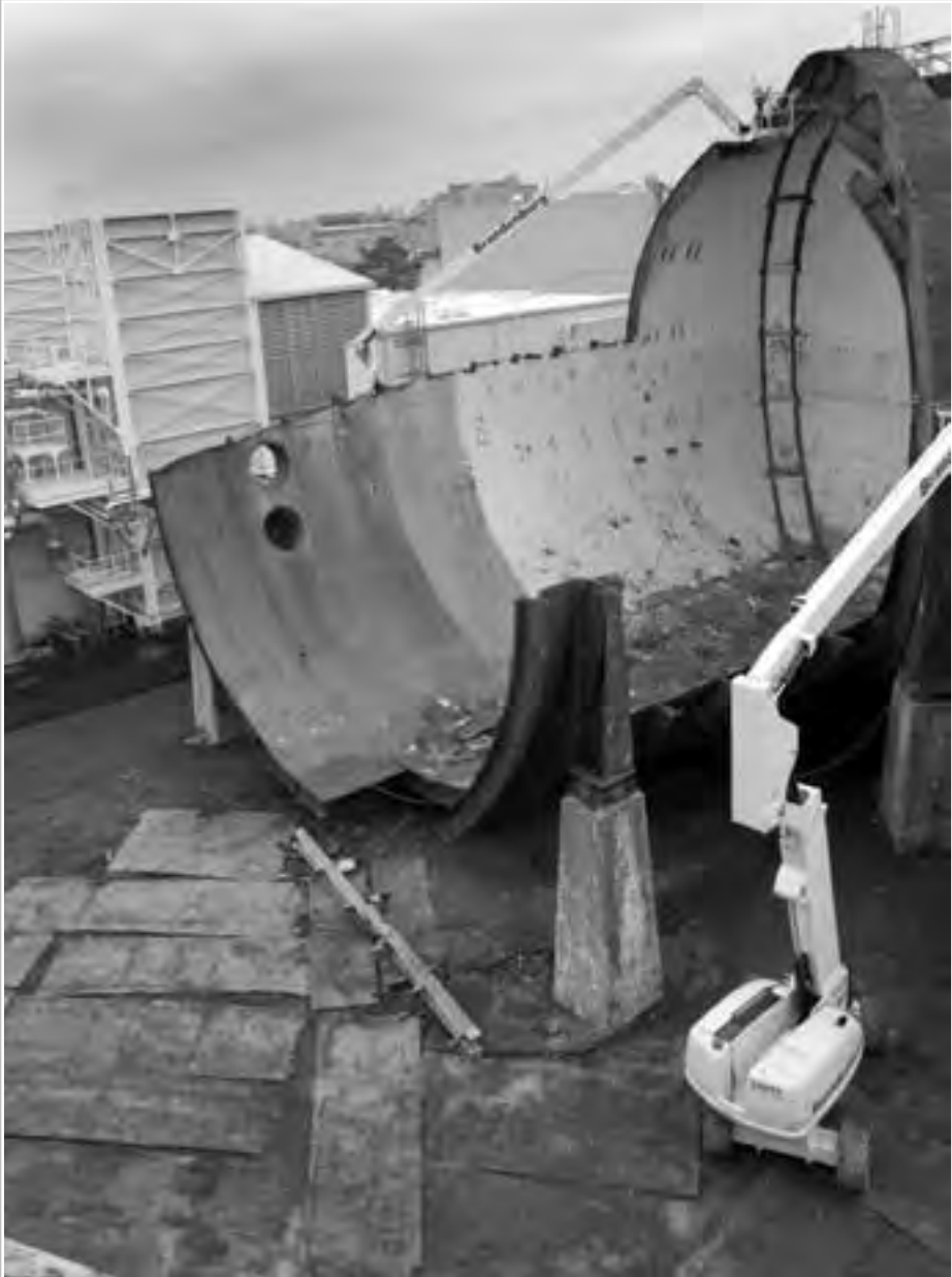
Image 290: As shown in this 26 February 2009 photograph, the removal of the structure started in the middle of the tunnel and proceeded to the two ends with their larger corner rings. Pieces of the shell were flattened and laid on the muddy ground to support the large cranes. (NASA C-2009-00752)
