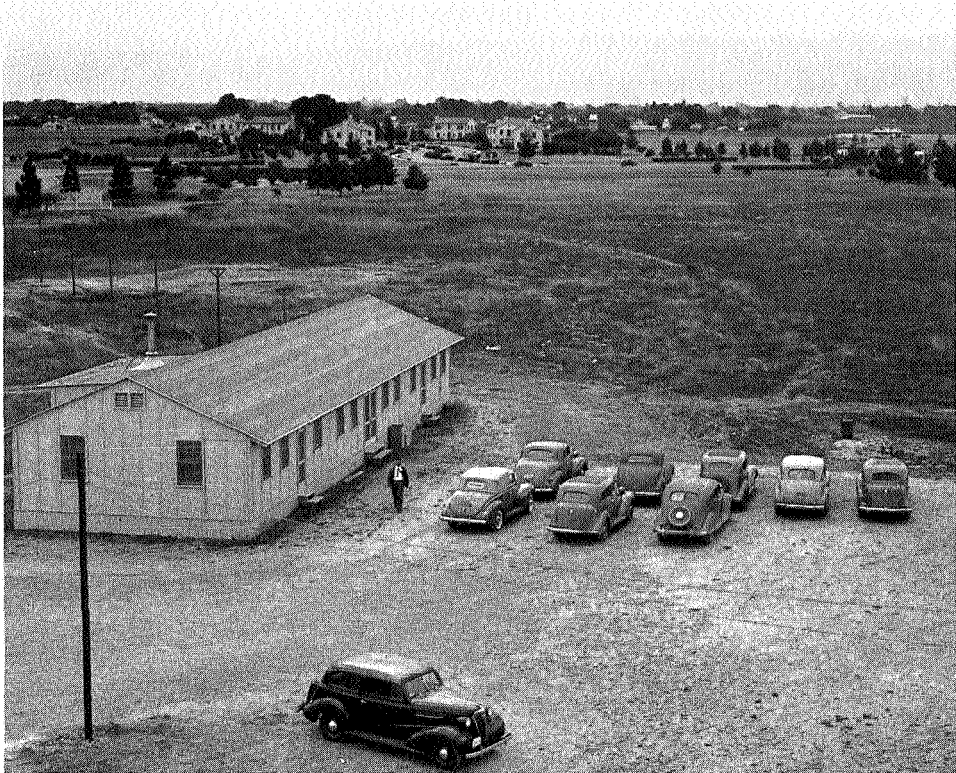
January 1940. The first building erected at Ames, the construction shack served as headquarters for the engineers and crews fighting California's winter mud as they laid out and built an aeronautical laboratory.
