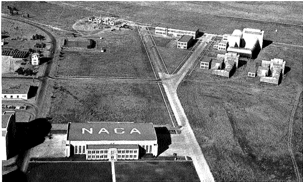
September 1941. After a year of operation, Ames boasted the Flight Research Laboratory (in foreground), two 7- by 10-foot wind tunnels, and behind them, a 16-foot tunnel. The field directly behind the center triangular plot would soon become the site of the 40- by 80-foot full-scale wind tunnel.
