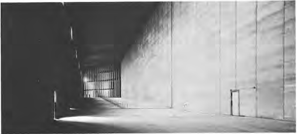
The view down the air-return passage in the Langley full-scale wind tunnel dwarfs two workers standing by the guide vanes. (LaRC)
