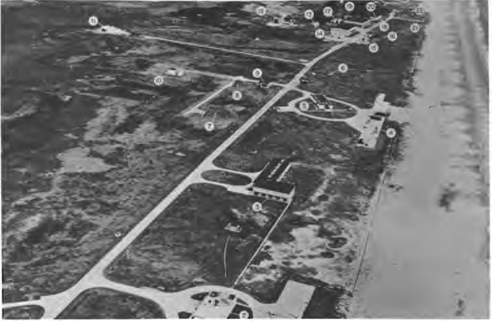
Aerial view of the Pilotless Aircraft Research Station, looking north along the Atlantic Ocean, in 1955. (LaRC)
