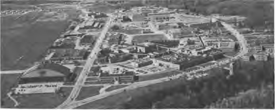
Aerial view of Lewis Flight Propulsion Laboratory as it appeared in 1955. An edge of the Cleveland municipal airport is visible at left center. (LeRC)
