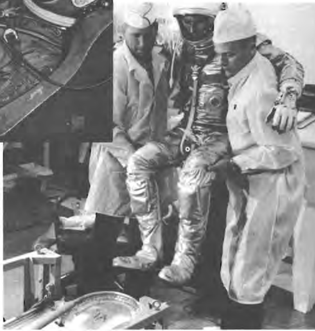
Astronauts had to learn to live with and operate in their life-support equipment. Above, Astronaut Shepard lies on a contour couch in his MC-IV pressure suit and practices navigation on the Langley Research Center simulator. Astronaut Cooper (right) is lifted in his pressure suit into a prototype net couch in Hangar S at Cape Canaveral, Florida.
