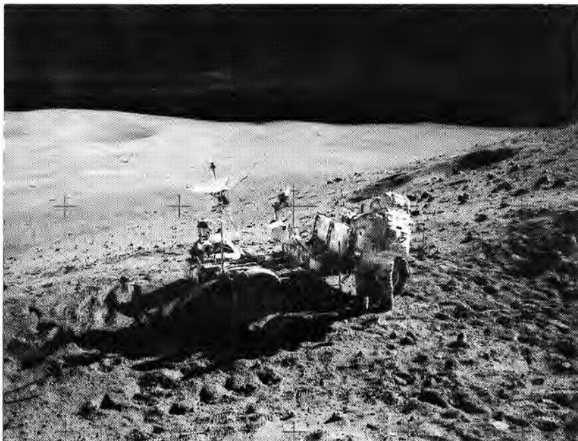
April 16-27: Astronaut John W. Young (above) walked away from the deployment site of the lunar surface experiments package during Apollo 16's first EVA April 21. Components in the background are central station, radioisotope thermoelectric generator, heat flow experiment, and lunar surface magnetometer. The lunar surface drill is at right center and its stems at left center. Below, Young—photographed by Charles M. Duke, Jr., while Thomas K. Mattingly II took lunar and astronomic photos from the command module in lunar orbit—replaced tools in the lunar roving vehicle beside Stone Mountain during EVA-2 April 22. Smokey Mountain is in the background.
