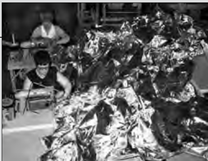
Two seamstresses stitch together a sunshade for the Skylab Orbital Workshop, the first U.S. experimental space station in orbit, which lost its thermal protection shield during the launch on 14 May 1973. (7040525)
