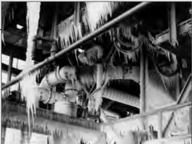
Ice on the pad on the day of STS-51L's launch. The ice caused the loss of elasticity in the SRB O-ring seals. (GPN-2004-00011)
