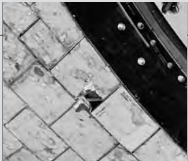
This thermal tile damage to one of the pods protecting Space Shuttle Endeavour's Orbital Maneuvering System occurred during STS-68. (STS068-067-013)
