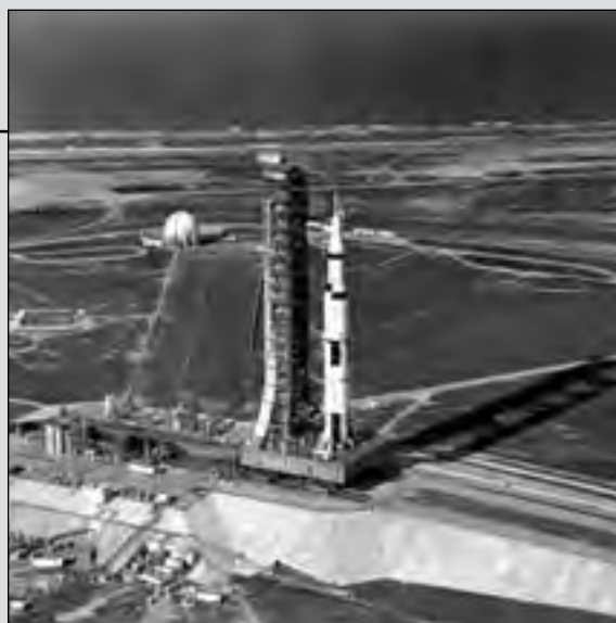
The Transporter nears the top of the 5-percent incline at Launch Complex 39A with the Apollo 11 Saturn V. (69P-0410)
