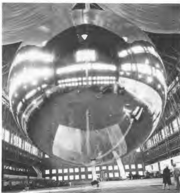
PAGESOS 1 inflation test, above, and a Pegasus satellite with wings outspread in an artist's drawing.
