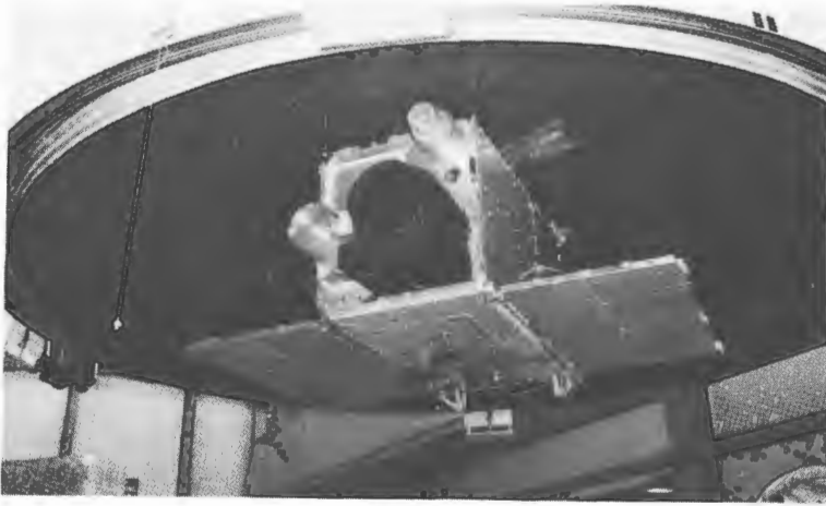
Structural model of TD-1A (above) showing the telescope, suspended for a space simulation test (ESC photo). At left, Telesat satellite Anik 1 in production (Hughes Aircraft Co. photo); below a composite photograph of the Telstar 1 spacecraft in space.
