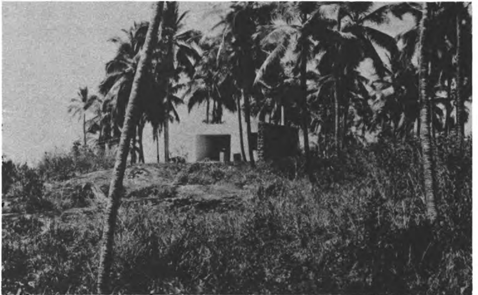
Static test stand for small experimental rocket motors at Thumba Space Sciences and Technology Center India.
