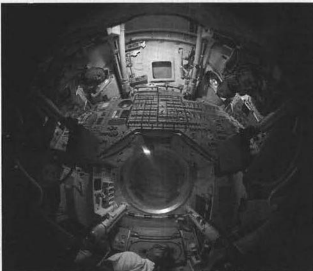
The command module mockup under construction by North American Aviation at Downey, California, shows the more spacious three-person interior of the Apollo spacecraft.
