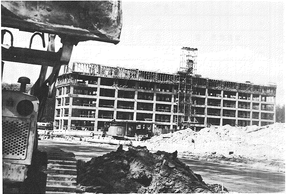
Building 8 under construction, July 1962.
