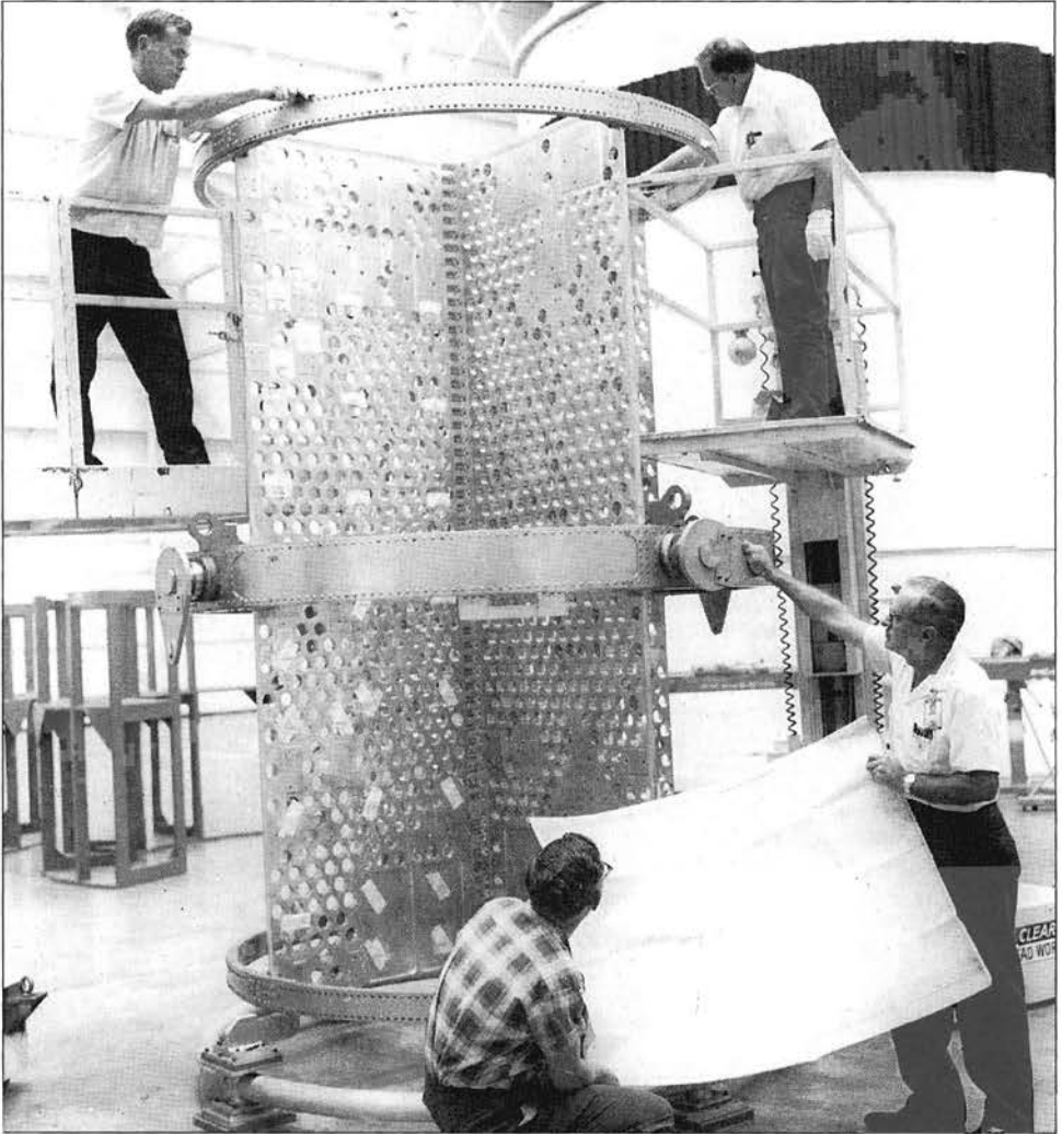
Technicians at work on a piece of test hardware for the Apollo Telescope Mount for Skylab at the NASA Marshall Space Flight Center. Called an ATM spar assembly, this piece of hardware was made for heat tests in a Marshall Center vacuum chamber. Replicas of the ATM solar experiments and other equipment were mounted on the spar and a metal outside covering added. The ATM canister was tested in MSFC's Sunspot II vacuum chamber. Working on the spar are, from the top left, Ronald Andrews and R.M. Freeman; J.B. Pendgraft, kneeling; and J.R. Clift, holding blueprint, all of the Manufacturing Engineering Laboratory. (NASA photo no. 69-H-1621).
