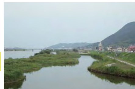
芦田川の植生浄化 Water Purification(Ashida River)
