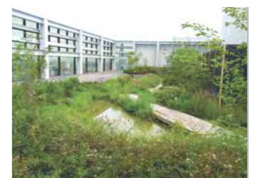
地上80mの屋上に生物多様性に配慮した空間を創出 (名古屋丸紅ビル) 80m aboveground, a space for biodiversity has been created on a roof. (Nagoya Marubeni Building)
