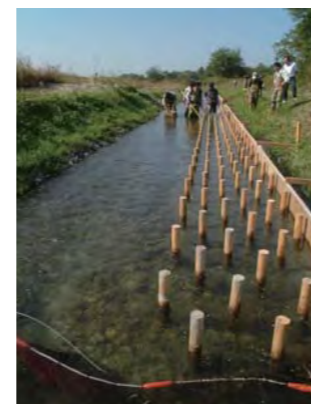
木杭群による魚類の生息場修復実験 Fish habitat restoration experiment using groups of wooden piles
