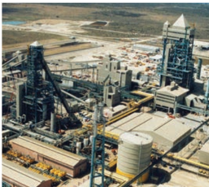
ArcelorMittal South Africa Plant COREX®/MXCOL®
