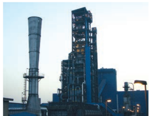
Hadeed Module E MIDREX® Plant, Saudi Arabia MIDREX NG™
