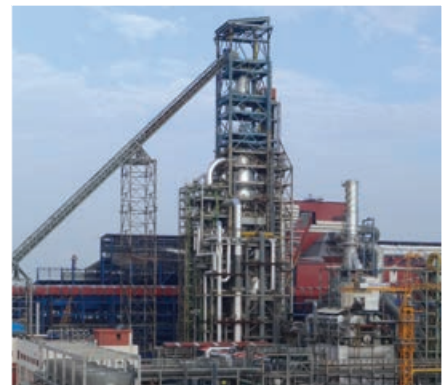
JSPL Angul I, India MXCOL® Coal Gasifier
