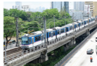
Manila Metro Rail Transit System Line 3 (MRT-3)
