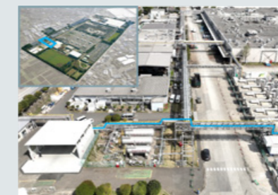
Hydrogen engine generator set demonstration facility
