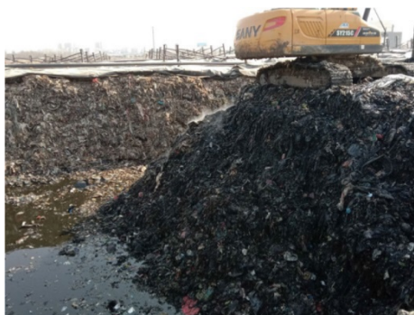
Figure 9 Excavation at the landfill site
