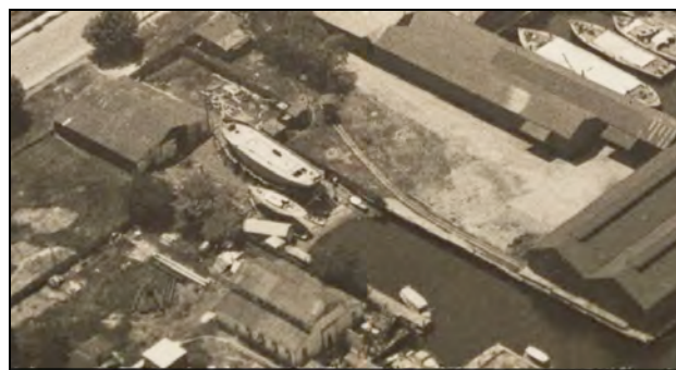
Aerial photo of Lawrence's yard taken by Fred Flood in 1932. The large vessel on the slips in front of Lawrence's shed (centre left) is the Silver Gull . Detail from photo BA2186/1-35 courtesy SLWA
