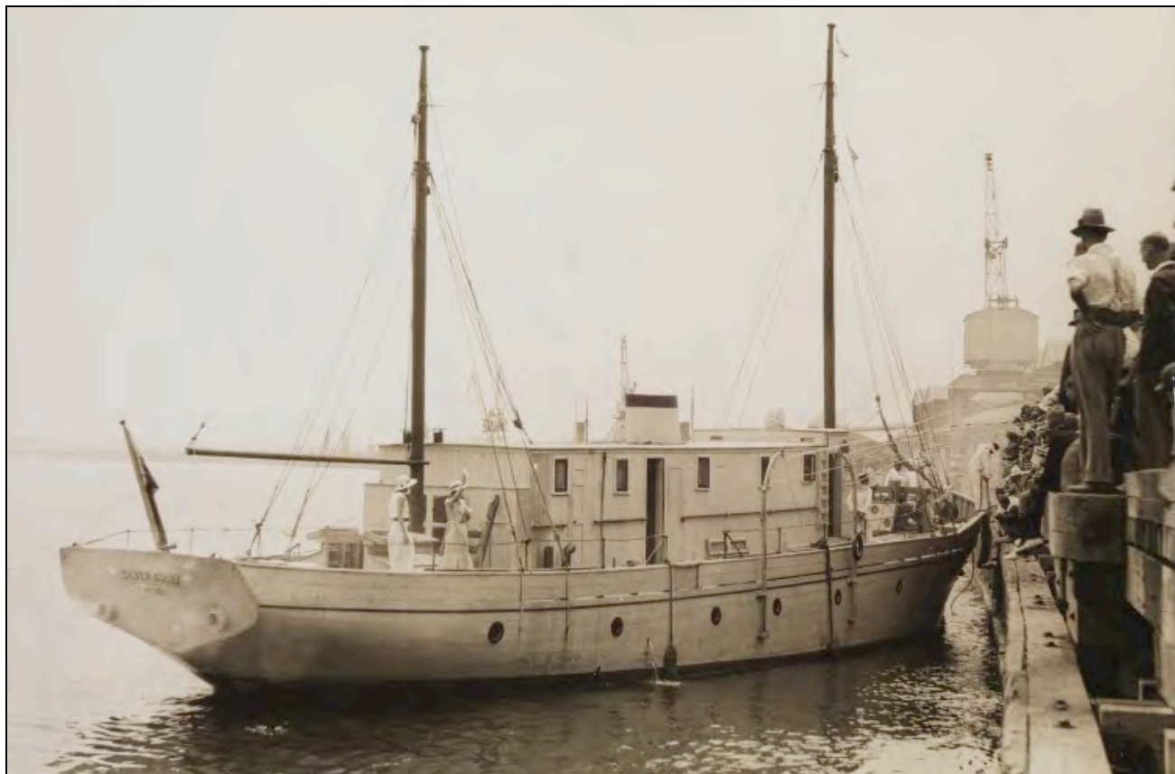
Photo by Frederick Flood of the auxiliary yacht Silver Gull making her departure from Fremantle 3 February 1934. The unsightly deckhouse was designed for easy removal after completion of the scientific cruises to allow the vessel to be turned into a South Sea island trader. The dummy funnel was actually a water tank. photo courtesy SLWA BA2186/96-115
