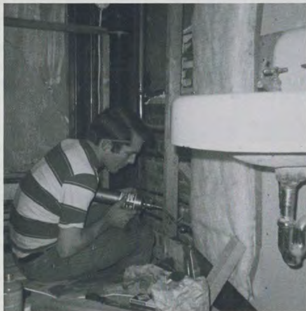
Colin S. Diver working on South End house, Boston, MA.
