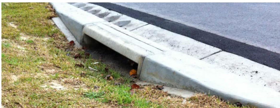
Figure 5-5 Concrete apron on grassed ZAM device avoids need for spray-strip or other edge management treatment. Source: 2018 ZAM-WSUD Handbook.
