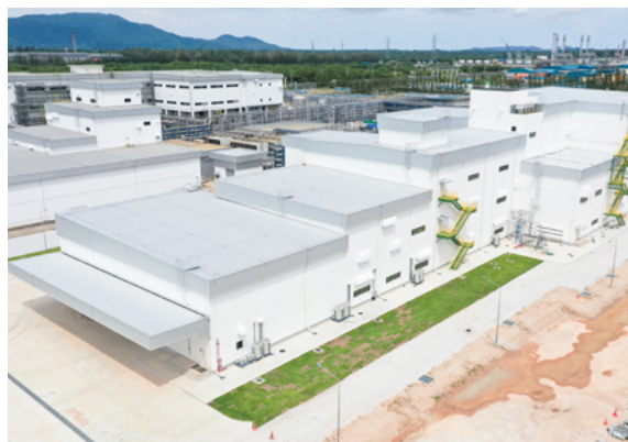
Thai Kyowa Biotechnologies' HMOs production facility
