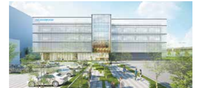
Image of new building at Value Creation Square (Head Office & Yokohama Business Center Area) (scheduled for completion in late summer 2024)
