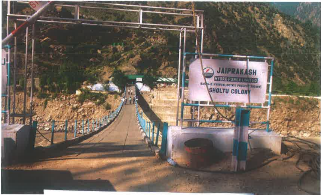
Photograph 1 - Ropeway Bridge at Sholtu Colony at Ch. 8.365 km
