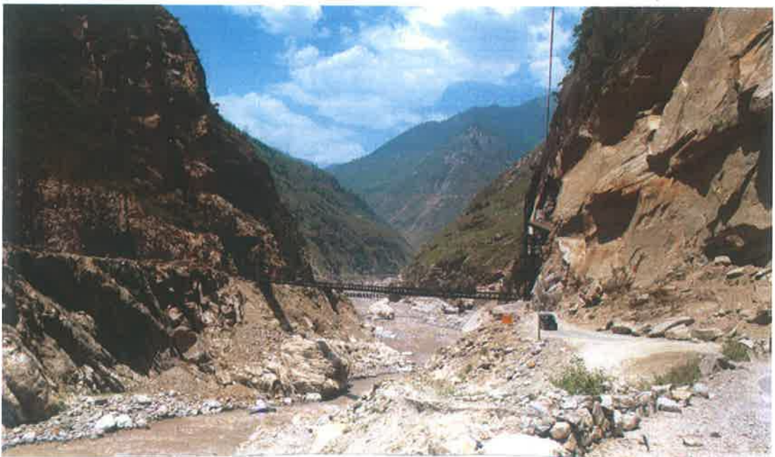
Photograph 2- 120.0 m Shatrujit Bridge at Ch. 18.317 km
