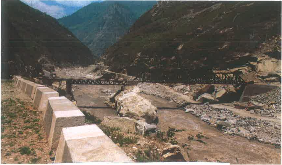
Photograph 3- 132.0 m Wangtoo Bridge at Ch. 18.677 km
