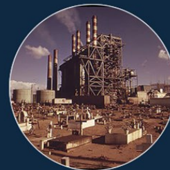
CRITICAL INFRASTRUCTURE MONITORING
