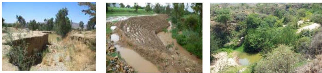
11 12 13 Figure 3.24 An example of how gullies are restored – the fully eroded gully (left) rehabilitated with vegetation 14 (center and right). Source: Alem et al. (2017)
