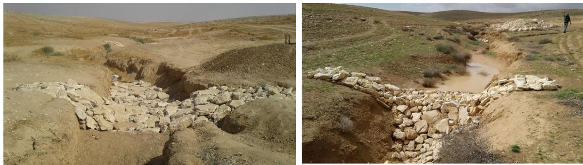
10 Figure 3.27 Gully plug development (September 2017) and post rainfall event in March 2018 11 near Amman, Jordan
