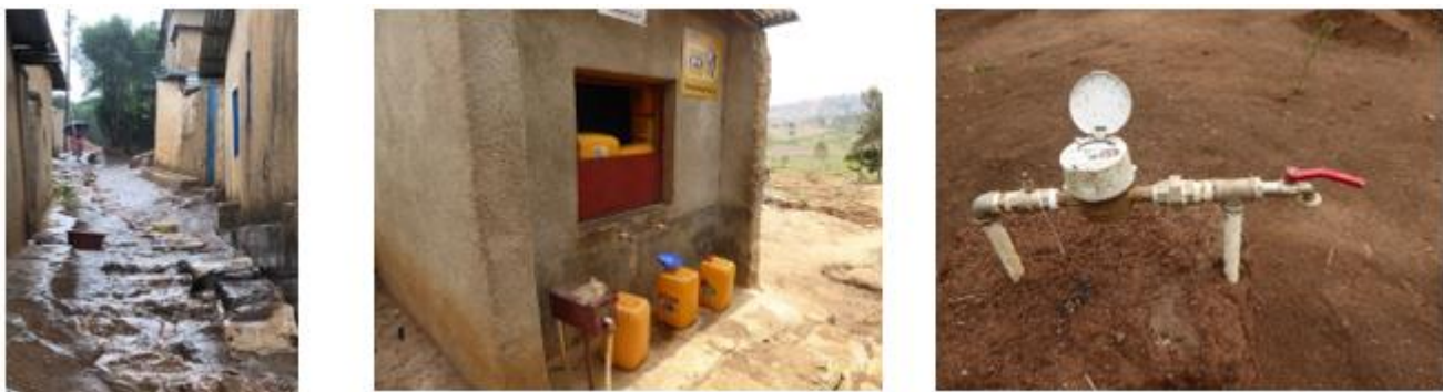
Figure 2: Rainwater harvesting from roof tops is common throughout the village. Water kiosk where residents can purchase water. A household water connection in the community
