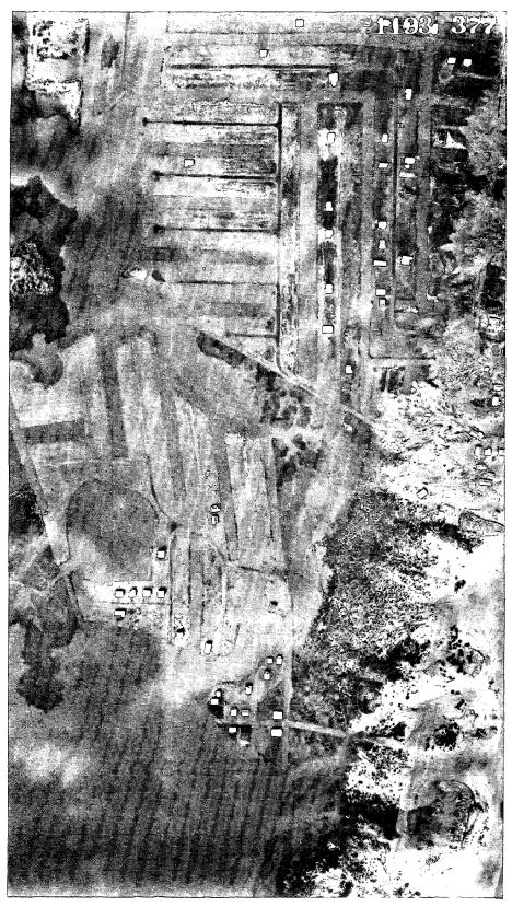
Photo 28 - Southern area of South Bethany, March 8, 1962. Notice the limited amount of development in 1962 and washover dunes from the ocean. This photo is an example of the series used for photo interpretation in preparing the storm damage map in this report.
