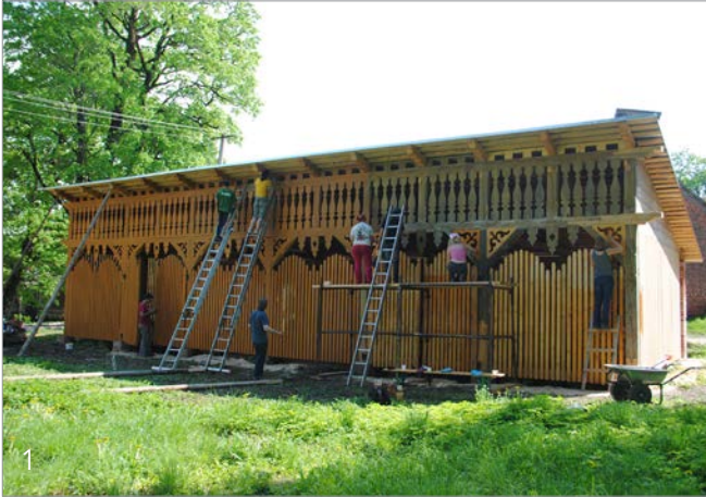
1. Painting a building at Loodi Manor with traditional paints, 2013. 2. Plastering course, 2012. 3. Restoring old windows, 2012. 4. Restoring granite walls in Vaida, 2014
