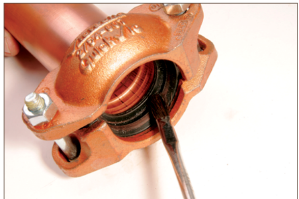
Figure 10.8. Applying lubrication to gasket
