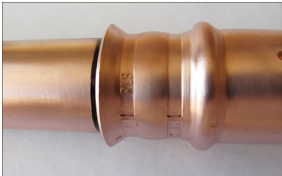
Figure 11.20. Press jaw crimp mark
