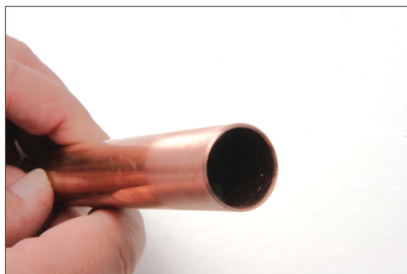
Figure 11.10. Properly prepare tube end
