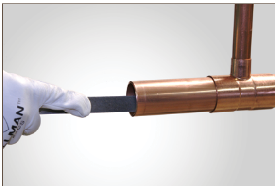
Figure 7.3. Reaming: File
