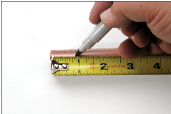
Figure 11.12. Measuring depth of insertion
