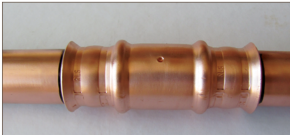
Figure 11.19. Completed joint with insertion marks visible
