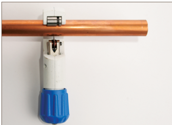
Figure 11.6. Cutting the tube square
