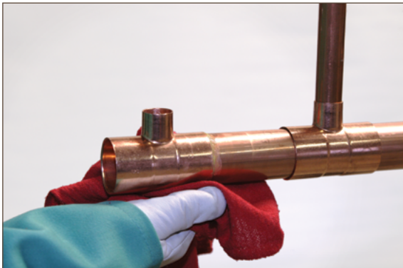
Figure 7.12. Removing Excess Flux
