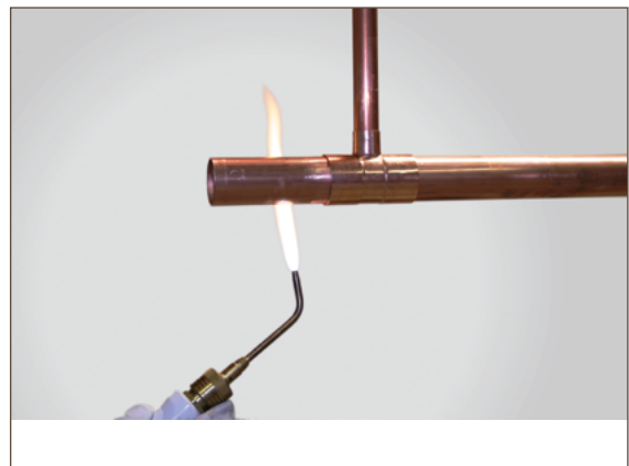
Figure 7.13. Preheating Tube
