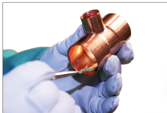
Figure 7.10. Fluxing: Fitting
