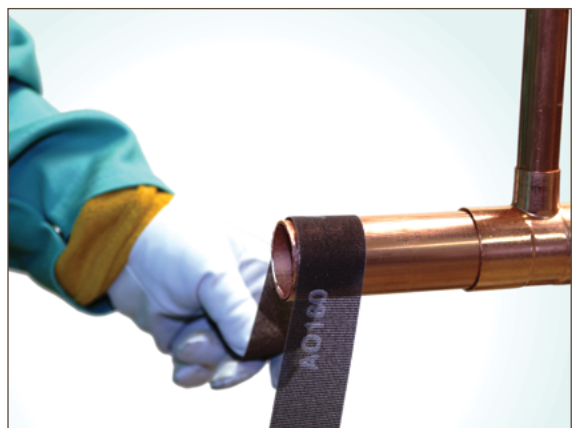
Figure 7.6. Cleaning: Sand Cloth
