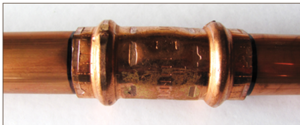
Figure 11.16. Completed installation of a press-connect joint
