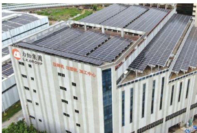
力勁集團最新的廠房已經安裝了太陽能板，採用太陽能發電，減低廠房運作時非再生能源的消耗量 LK Group’s newest plant is equipped with solar panels to provide solar power and reduce consumption of electricity from non-renewable sources
