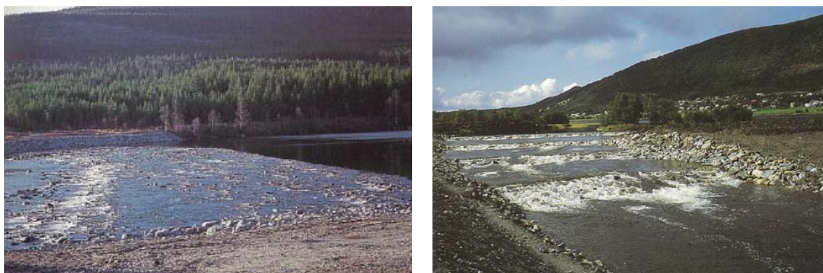
Figure 21. Groundsill made of loose material in the river Glomma near Lyngen (Hedmark district, left) and a series of small stone weirs in the river Hareidselv (Møre and Romsdal district, right). From Sæterbø et al. (1998)
